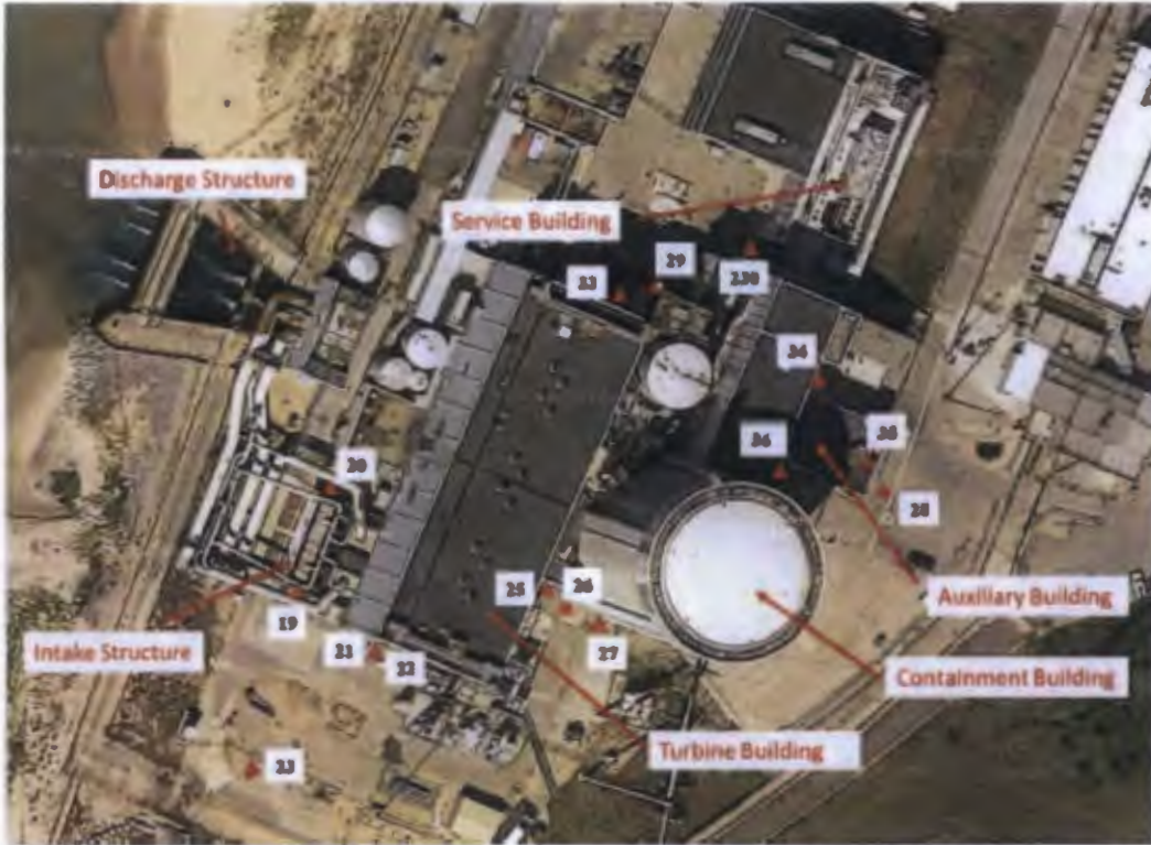
Figure 3.0-1 Palisades Site Layout (Adapted from Figure 3.2-1 of March 11, 2015, FHRR (ADAMS Accession No. ML15114A209)
