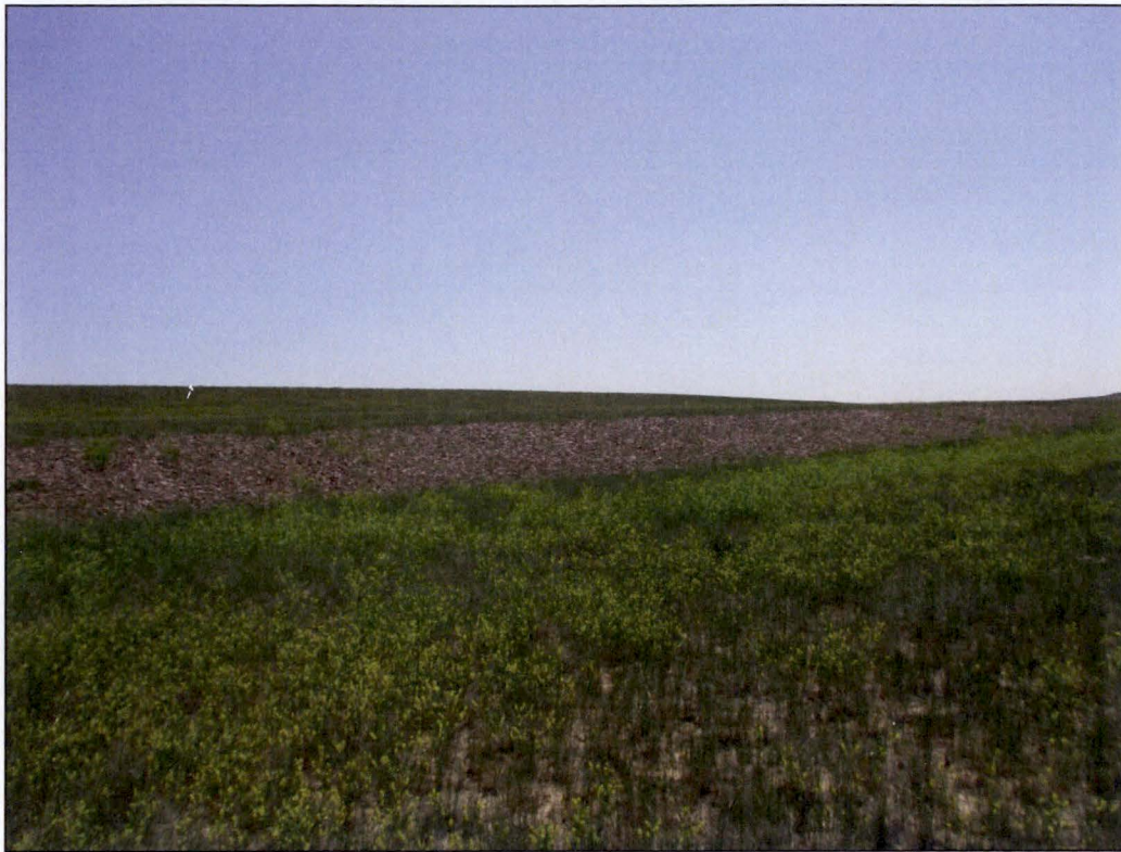
PL-9. Riprap-Armored Dam Outslope of Disposal Cell
