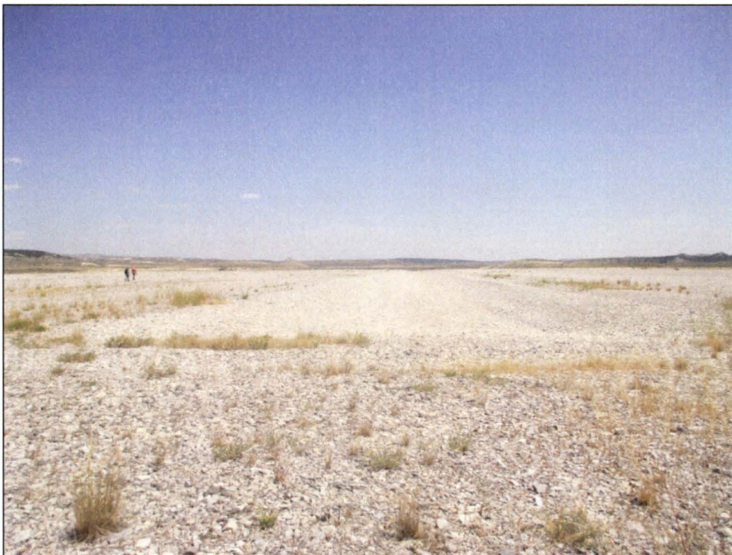
PL-8. Diversion Channel No. 1 on Top of Disposal Cell
