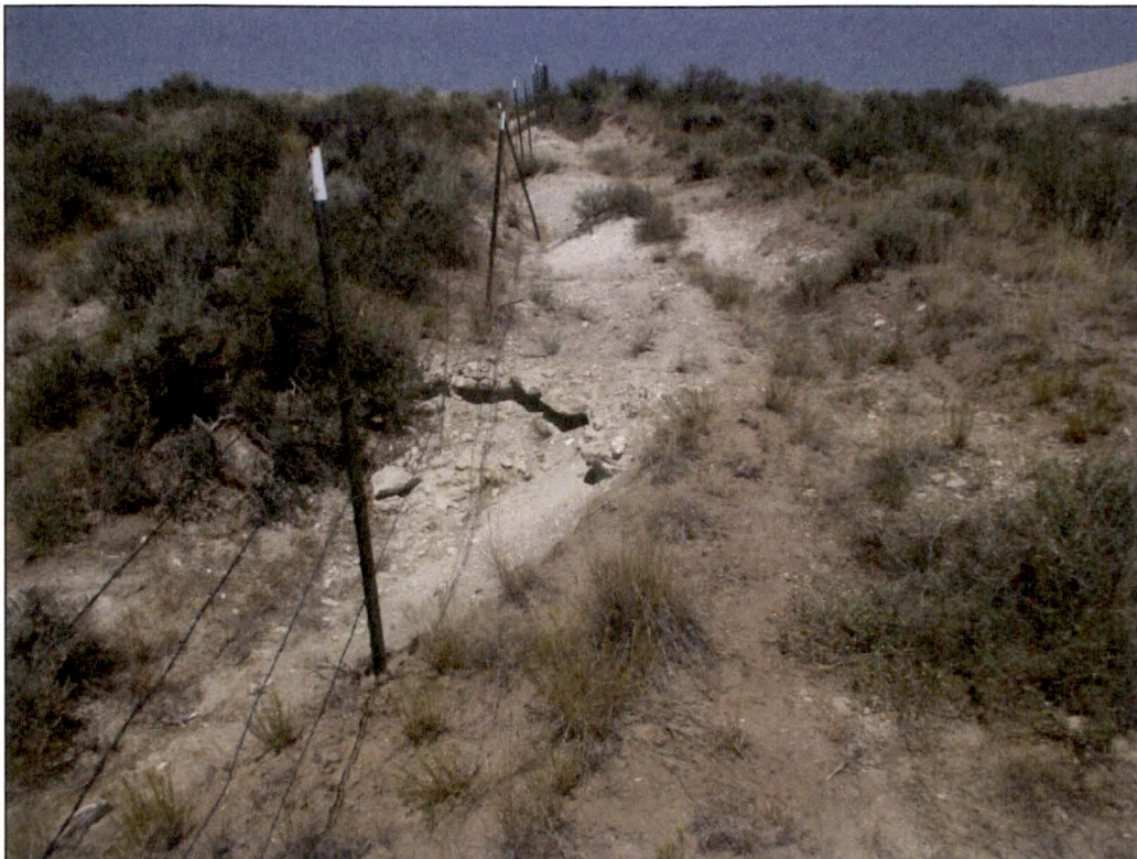
PL-1. Erosion Near Southwest Corner of Perimeter Fence
