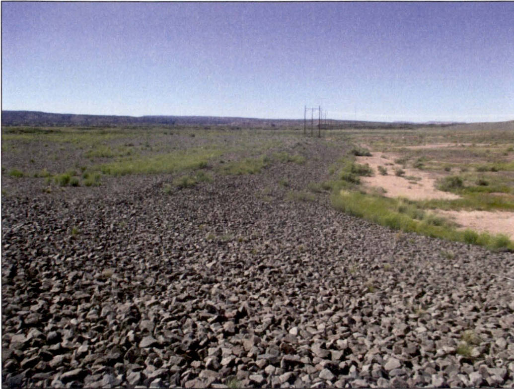
PL-11. Northeastern Side Slope of Northwestern Extension of Carbonate Tailings Cell
