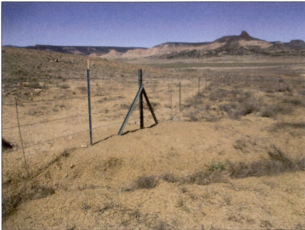
PL-1. Loose Fence Post Repair South of Perimeter Sign P33
