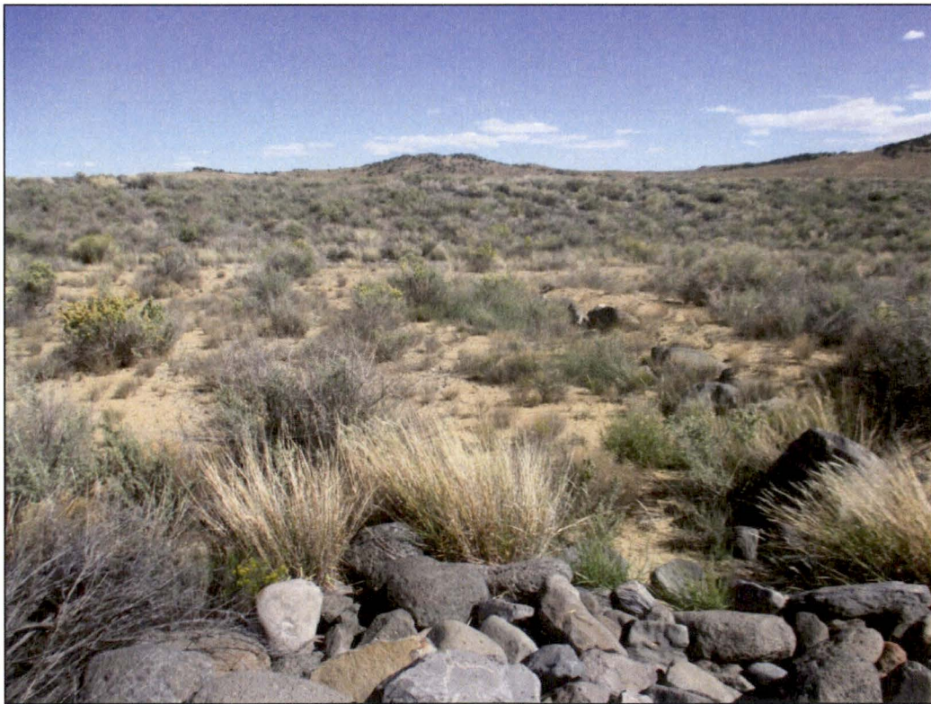
PL-18. Riprap Cutoff Wall at Outlet of North Channel and Disposal Cell Western Side Slope
