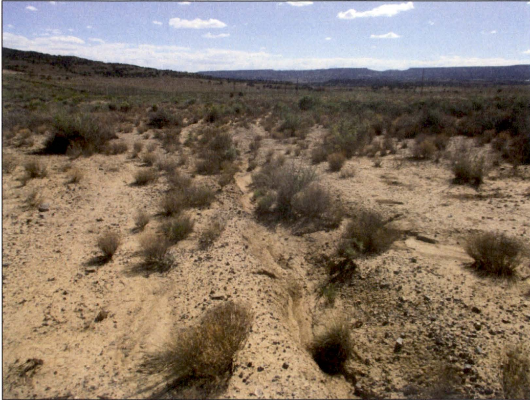
PL-17. Erosion East of Riprap Cutoff Wall at Outlet of North Channel
