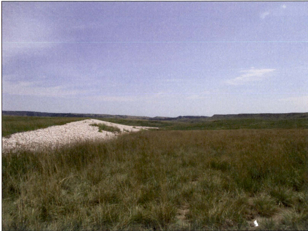
PL-11. West Portion of Containment Dam
