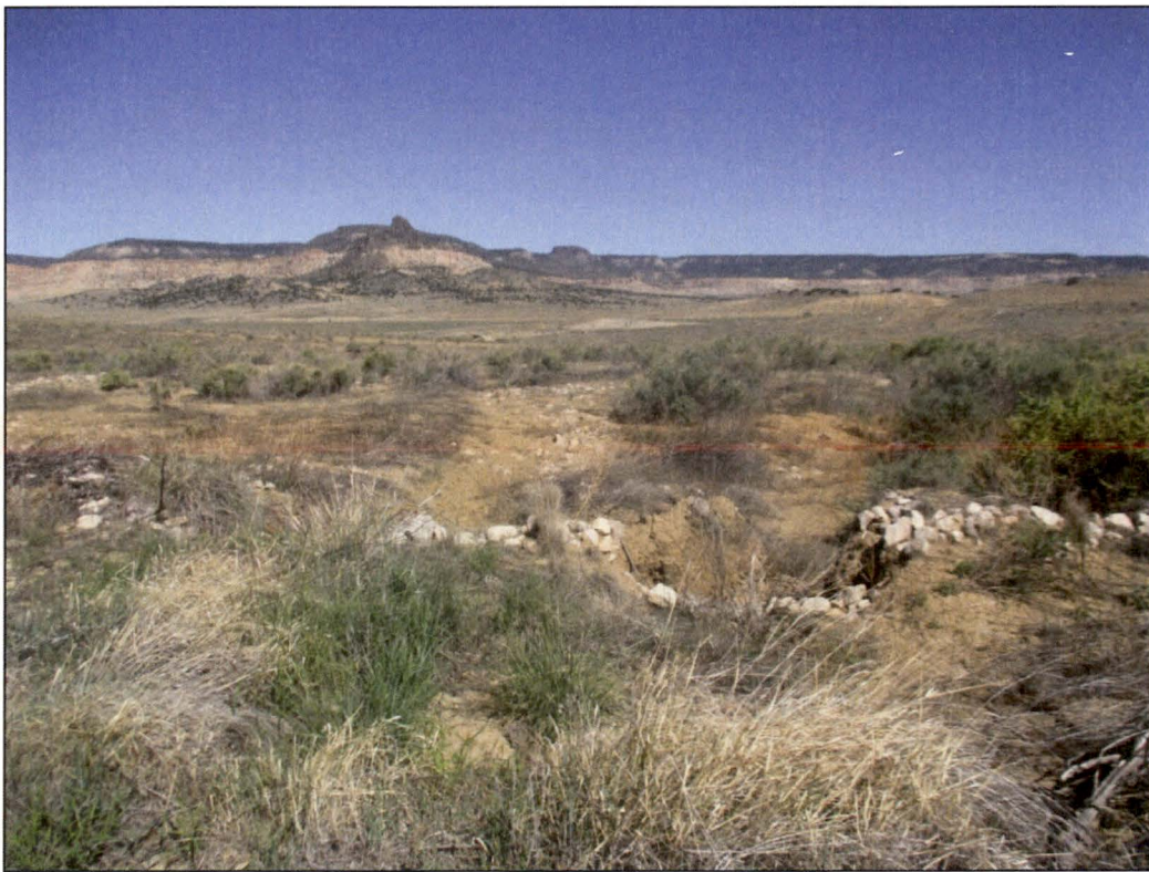
PL-12. Breach of Runoff Control Structure A Berm
