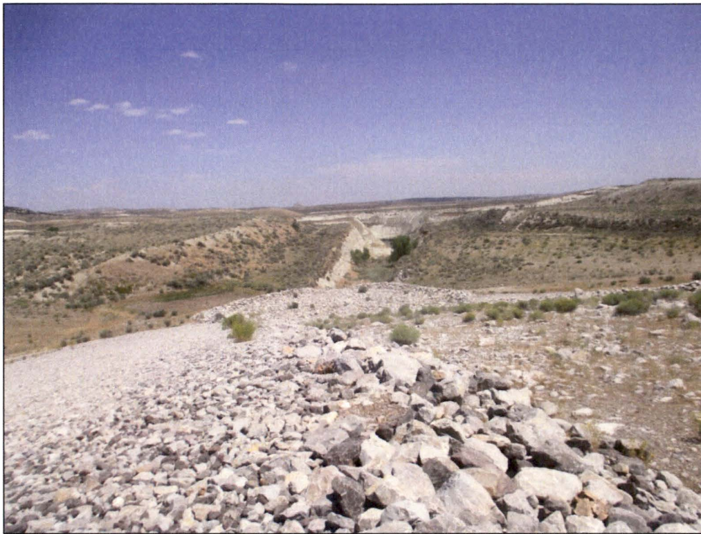
PL-15. Diversion Channel No. 1 Outlet on East Side Slope; Launch Rock Erosion Protection Basin and Rob Pit in Background
