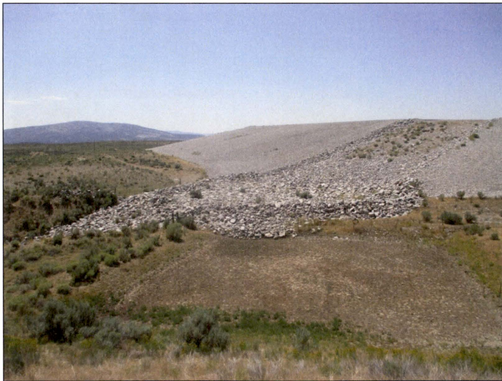
PL-14. Diversion Channel No. 1 Outlet and East Side Slope; Launch Rock Erosion Protection Basin
