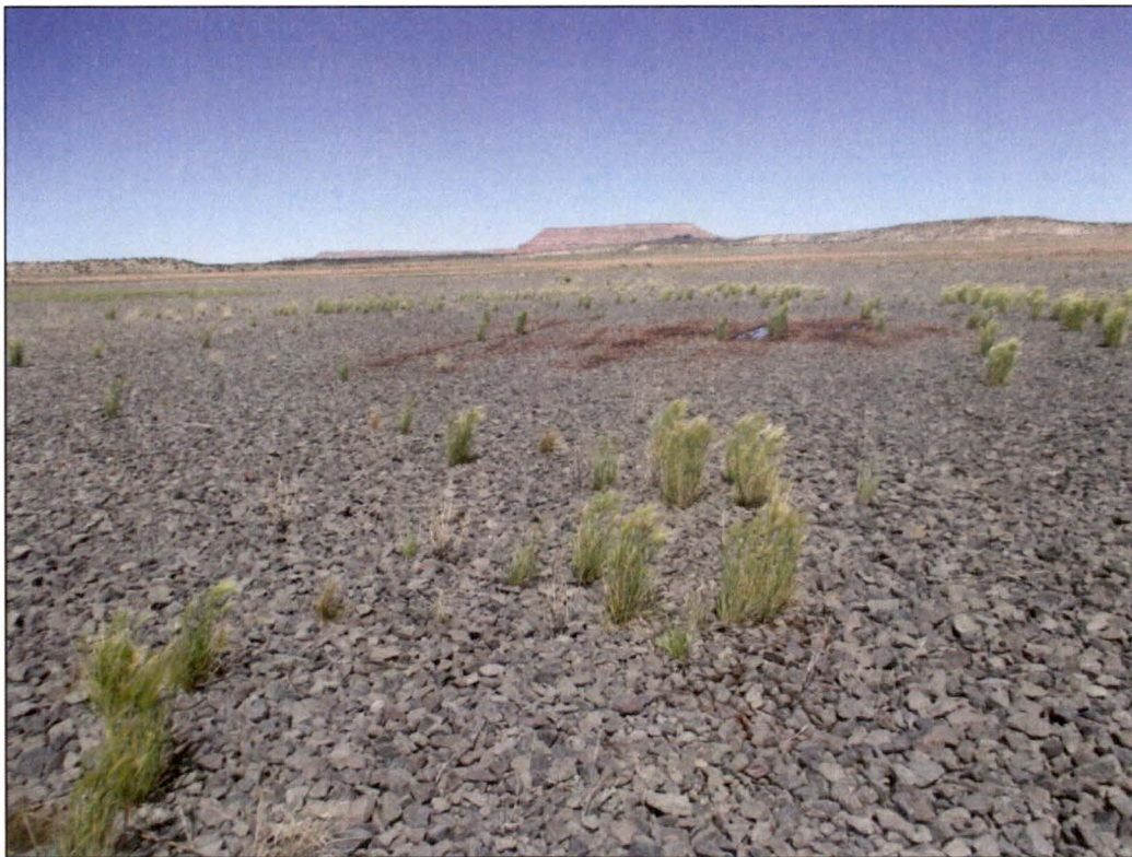
PL-8. Ponded Water on Main Tailings Disposal Cell Top Slope
