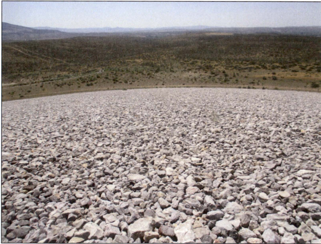
PL-10. Intersection of Disposal Cell's South and West Side Slopes
