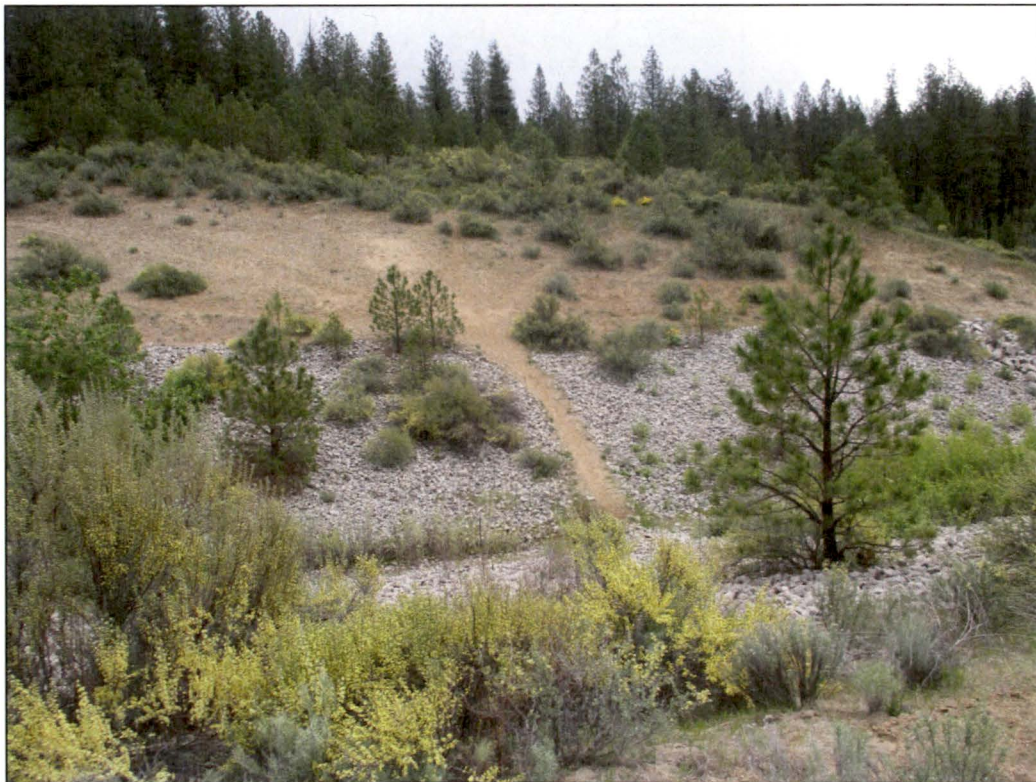
PL-10. Protective Rock Armor Displaced by Animal Trails
