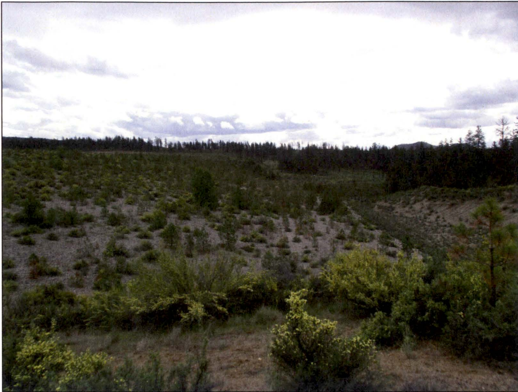
PL-7. Containment Dam Outslope
