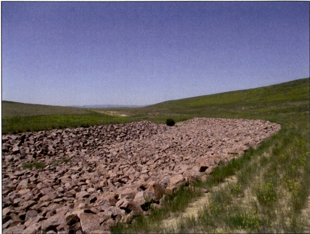
PL-11. Downgradient View of Riprap-Armored Portion of North Channel
