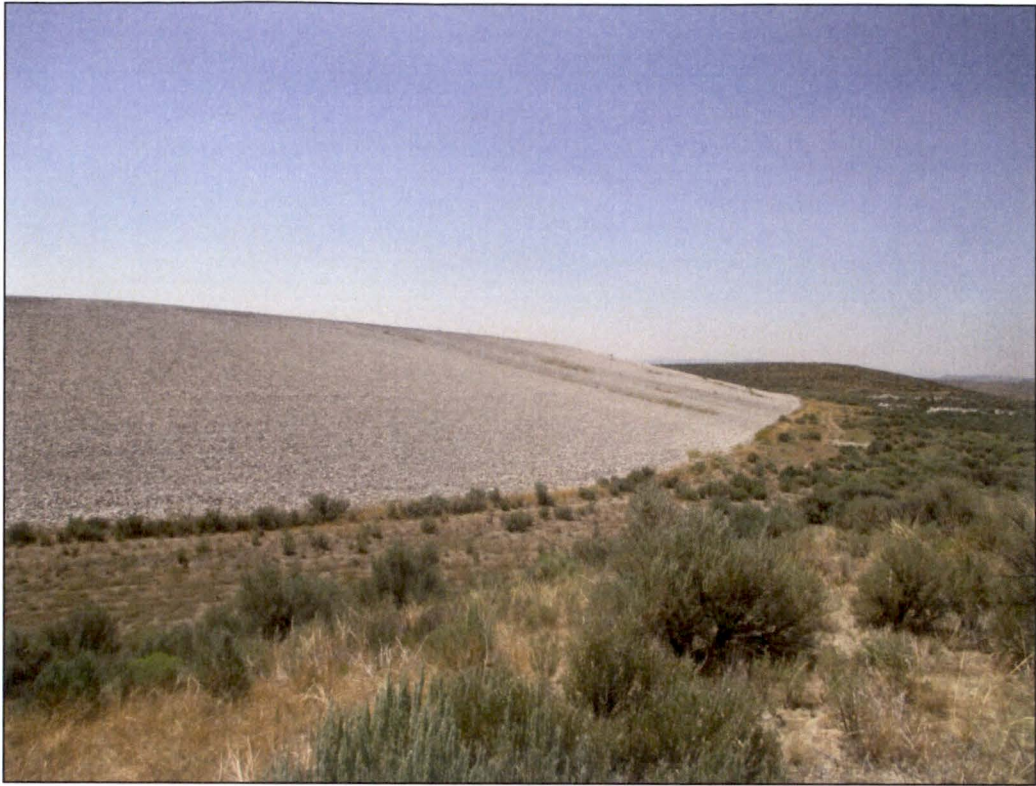
PL-9. Disposal Cell North Side Slope
