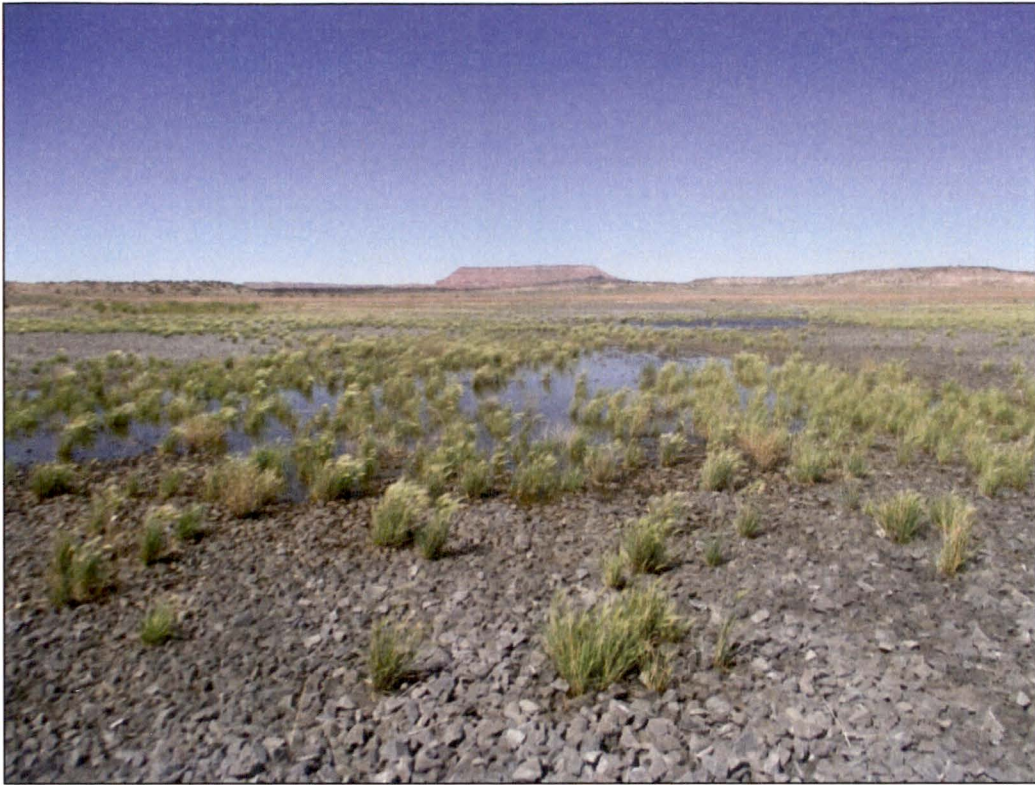
PL-7. Ponded Water on Main Tailings Disposal Cell Top Slope
