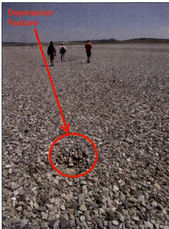
PL-7. Depression No. 3 on Top Slope of Disposal Cell
