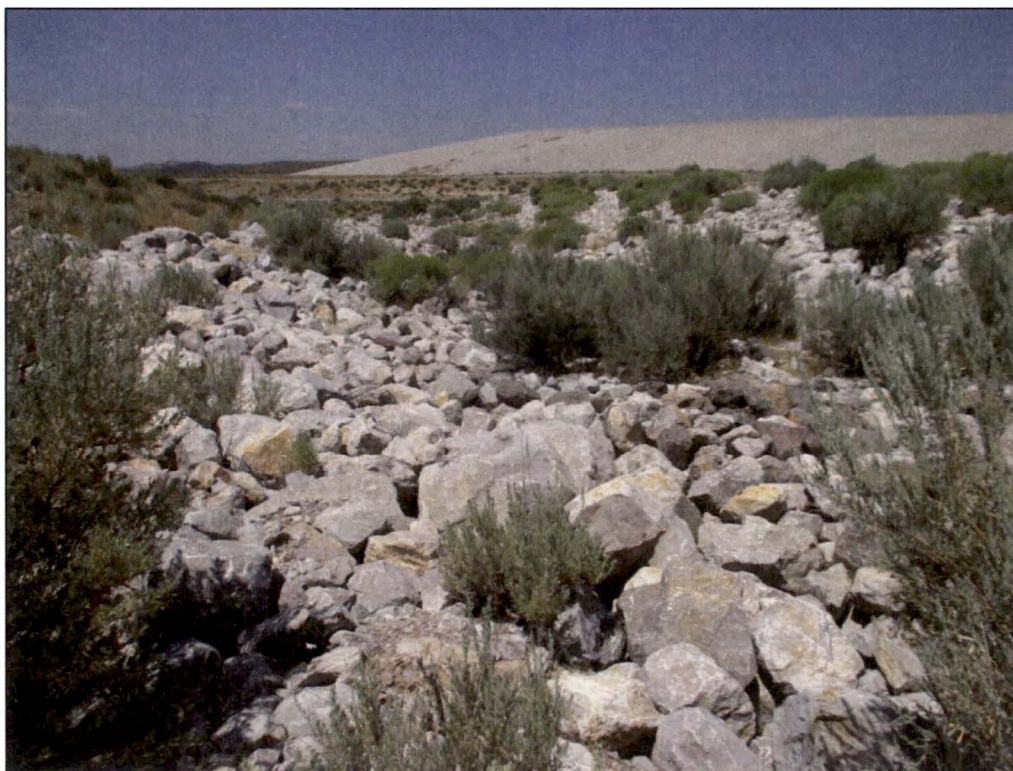
PL-16. Diversion Channel No. 2
