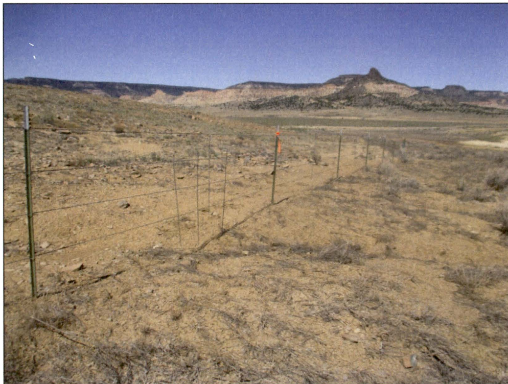
PL-2. Erosion Under Perimeter Fence and Fence Repair
