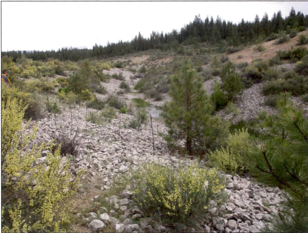
PL-9. Vegetation in East Diversion Channel
