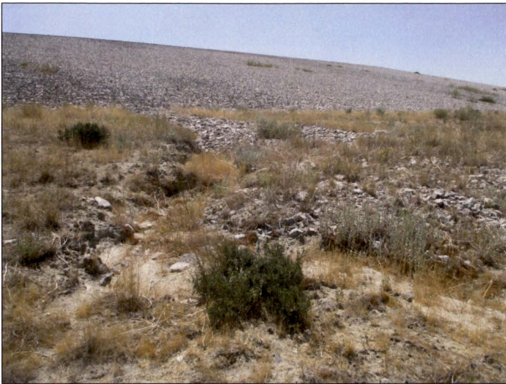
PL-11. Toe Drain on Disposal Cell North Side Slope and Adjacent Erosion
