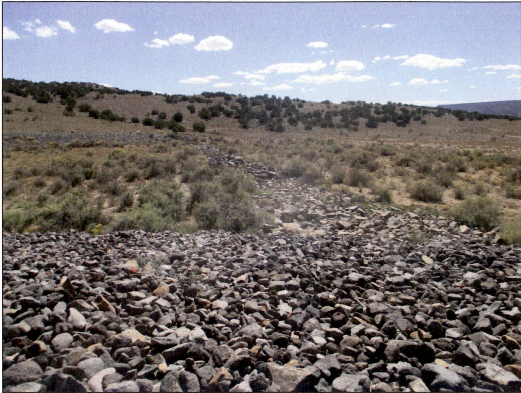
PL-21. Riprap Cutoff Wall at Outlet of South Channel
