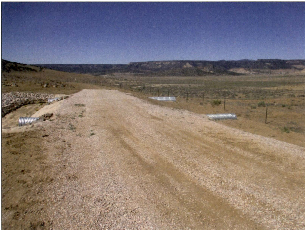
PL-22. Culverts Constructed in 2016
