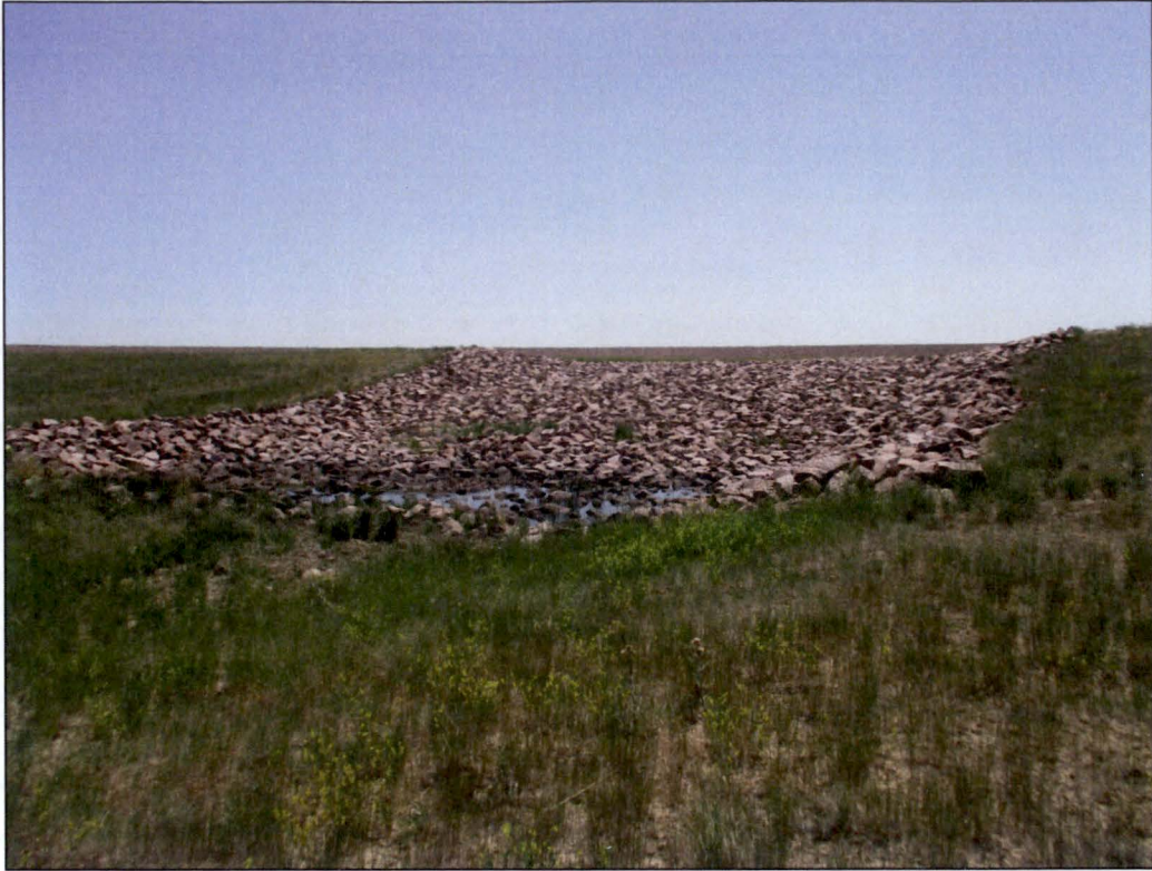
PL-7. North Swale Discharge Point
