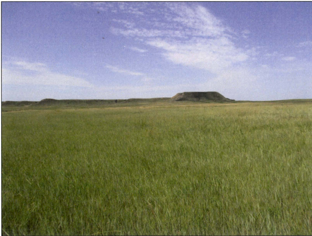
PL-10. Southeast Portion of Disposal Cell
