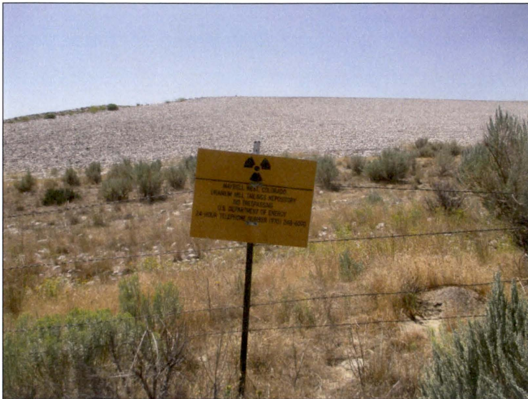
PL-3. Perimeter Sign P2; Disposal Cell Northeast Side Slope in Background
