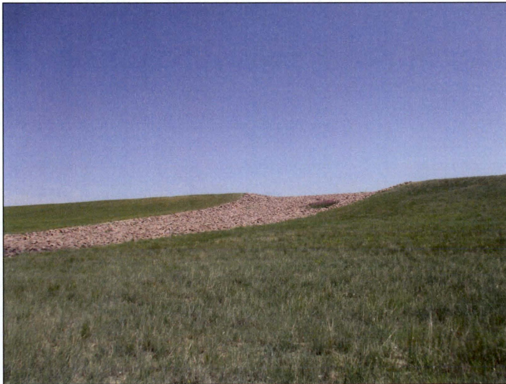
PL-8. South Swale Discharge Point
