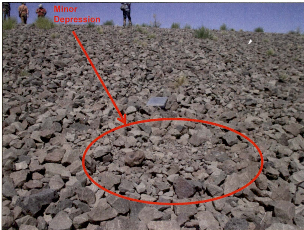
PL-10. Minor Depression on Main Tailings Disposal Cell South Side Slope
