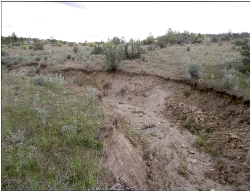
PL-4. Gully Outside Site Boundary near Perimeter Sign P1
