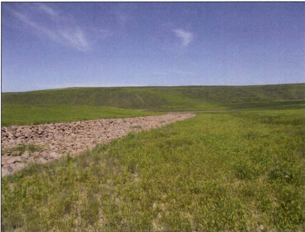
PL-10. Upgradient View of Riprap-Armored Portion of Southwest Channel
