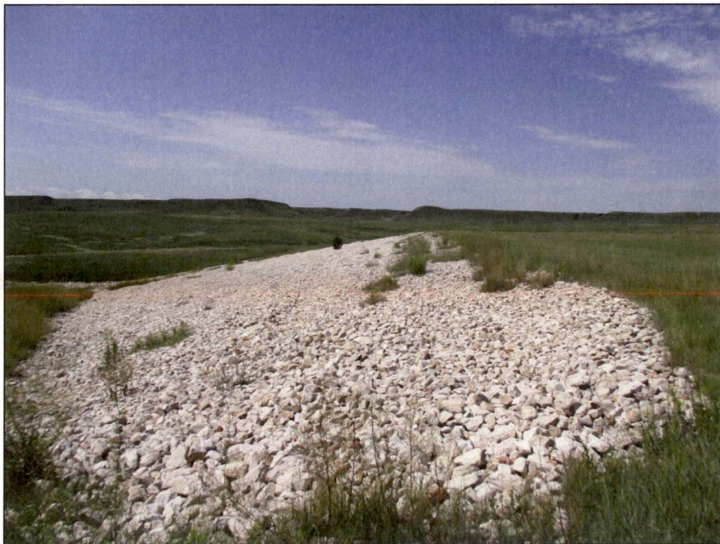
PL-12. East Portion of Containment Dam
