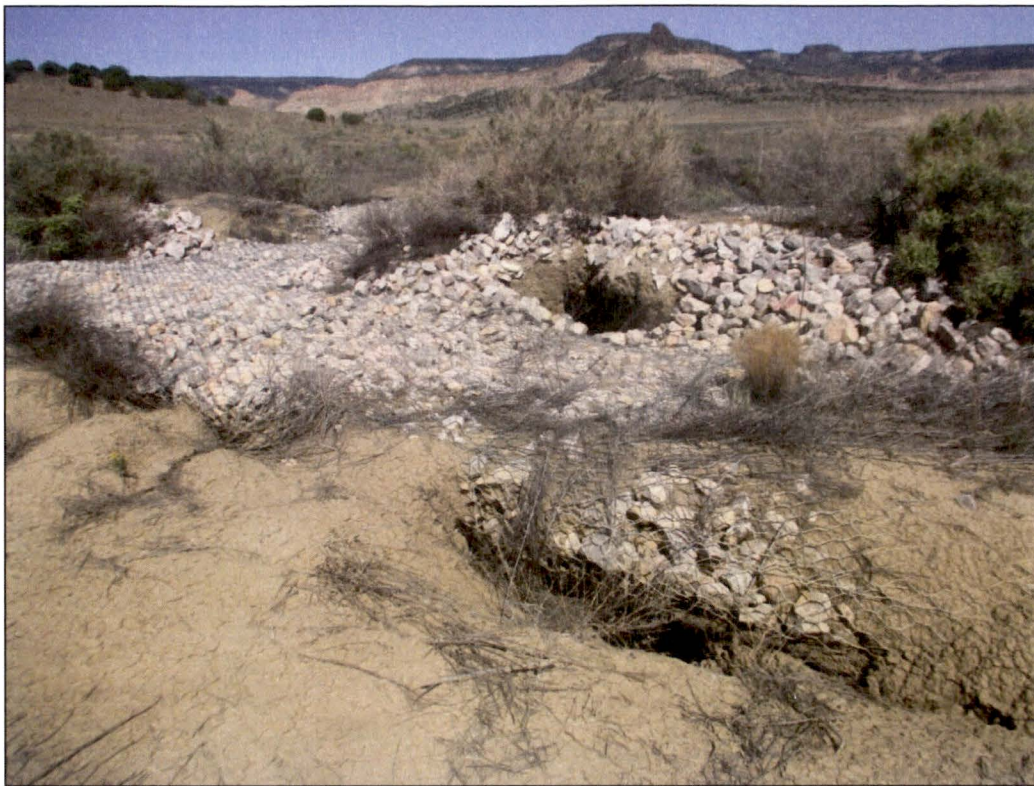
PL-13. Soil Piping Along Inlet of Runoff Control Structure A
