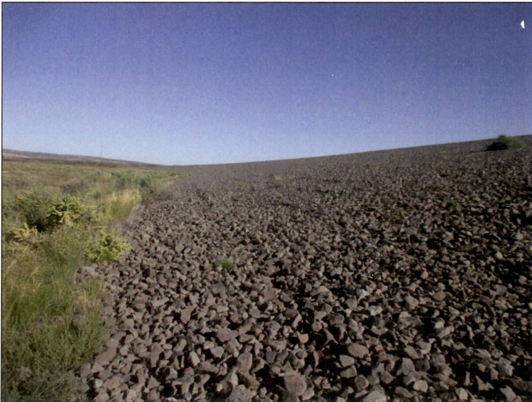
PL-6. South West Side Slope of the Main Tailings Disposal Cell
