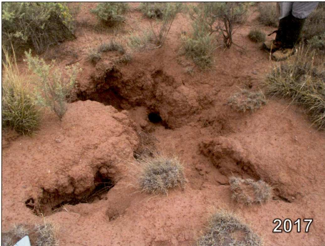
PL-17. (b) Settlement on Soil Cover of Disposal Area No. 1—2017 (Photo for Comparison)
