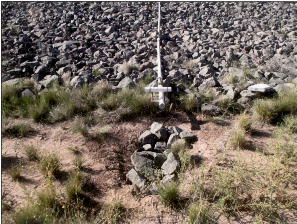
PL-9. Outlet of Siphon at Toe of Main Tailings Disposal Cell
