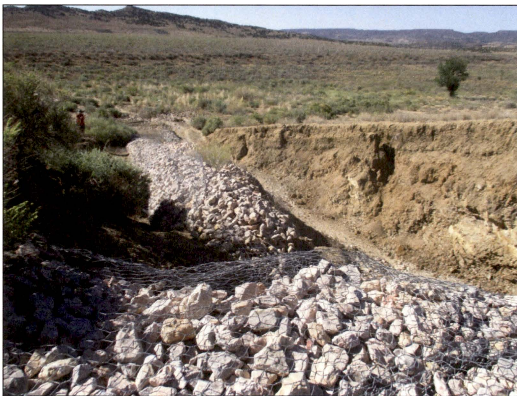
PL-16. Damaged Runoff Control Structure G
