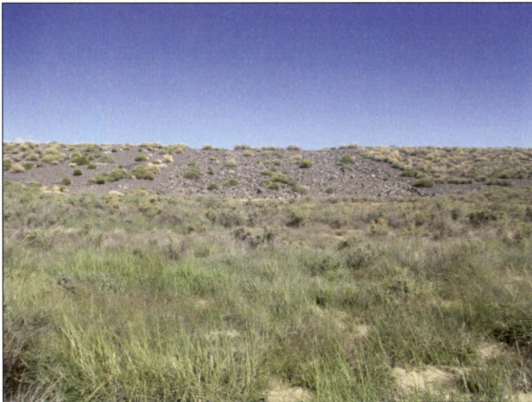
PL-10. Containment Dam Spillway
