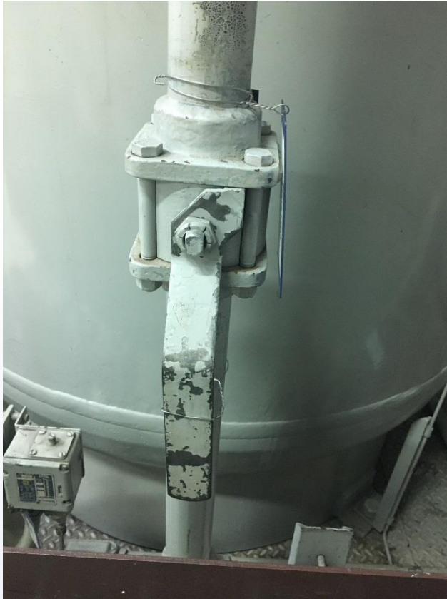
Division 2 DG air start valve in the normal "Locked Open" position
