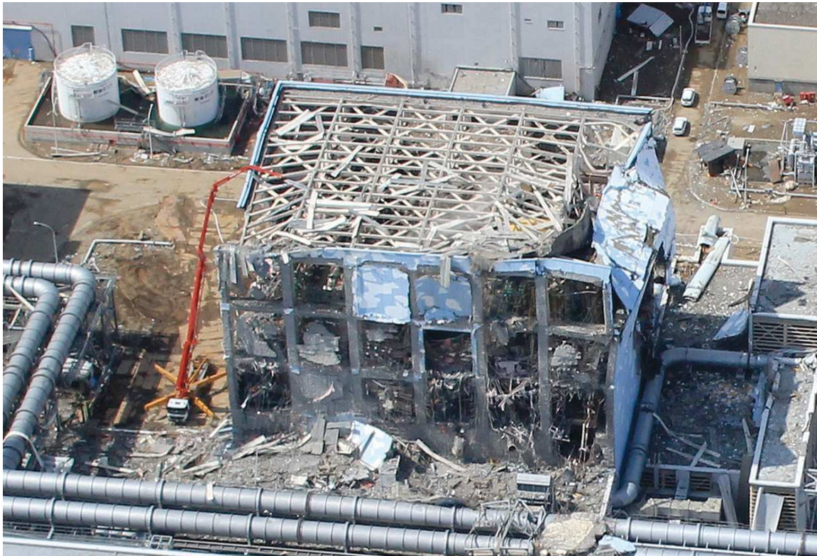
Figure VIII-1 Unit 4 at the Fukushima #1 Site During the 2011 Accident
