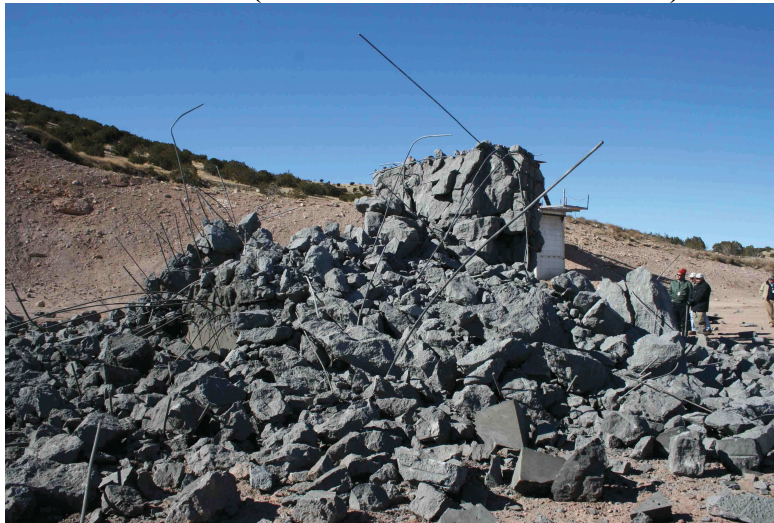
After Test (viewed from the attacked face)
