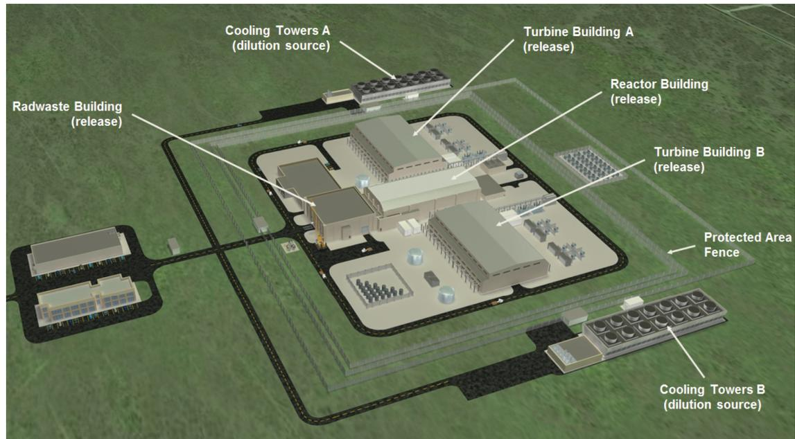
Figure 2-1 NuScale plant layout with release points identified
