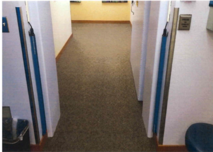
Figure 1 - HDR Treatment Room access with the laser curtain sensors in blue.
