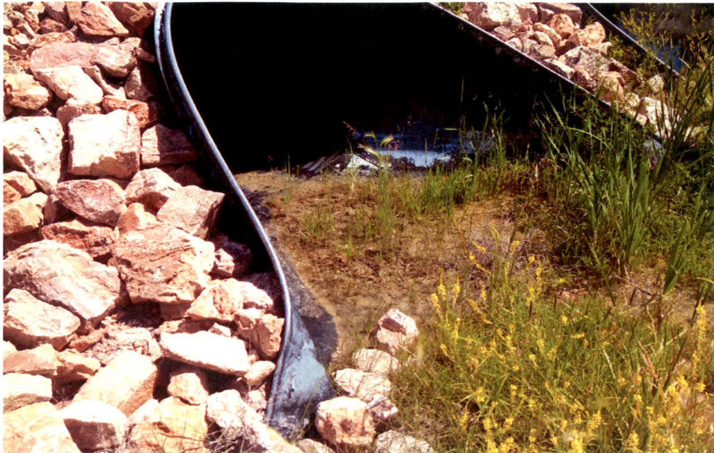
Grass and Sediment in the Outlet of the Diversion Culvert
