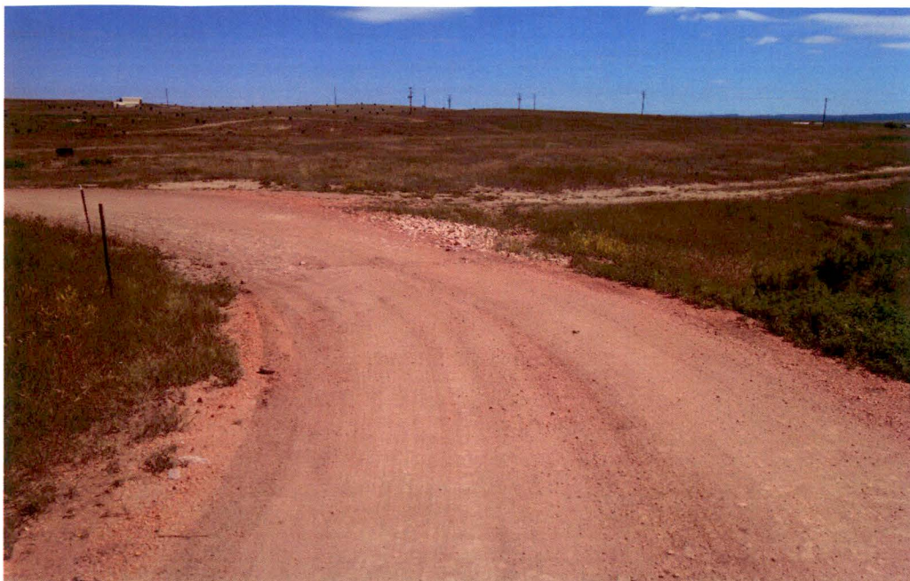
Silted Riprap at the Road Crossing of the Emergency Spillway
