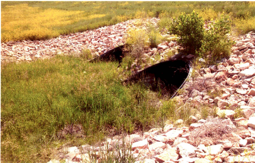
Shrub on Top of the Outlet of the Diversion Culvert
