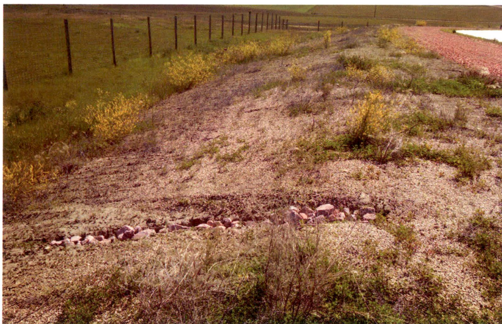
Repaired Gullies on North Side of Cell 3
