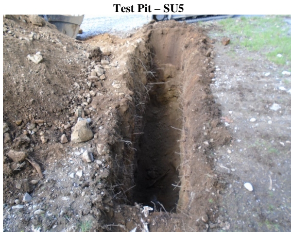
The background soil is relatively free of large rocks and it is laid in layers, which appears natural.
