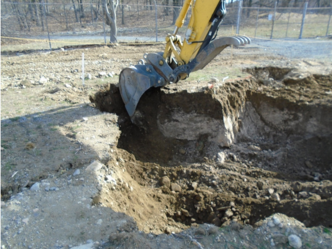
Figure 2-5. Buried Contamination found in SU2
