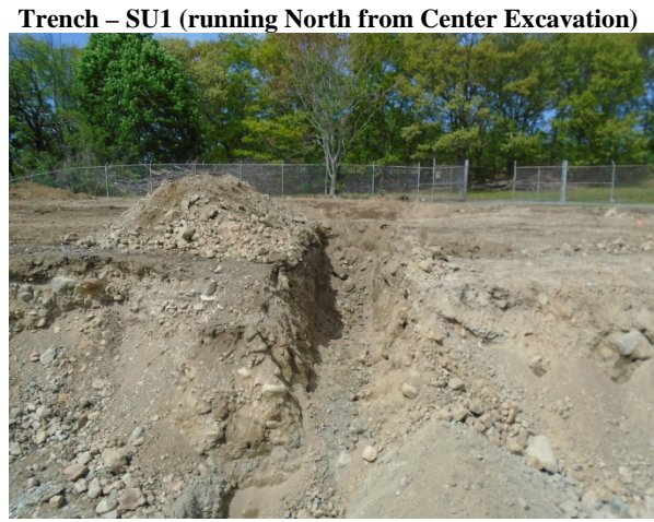
Typical of the impacted area, soil is a mix of sand, soil, rocks, and boulders. This appeared to be backfill material.
