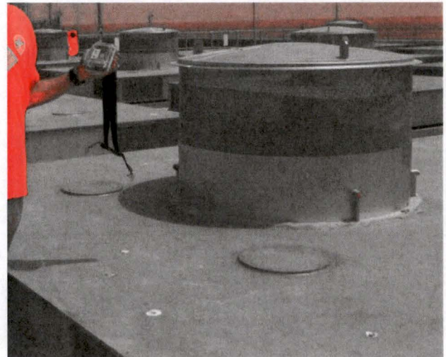
Holtec UMAX lids with large air vents. Round top has outlet air vent. Lower rectangular part of lid has inlet air vents near all corners. Radiation reading at San Onofre were 324 CPM (counts per minute) with no leaks in canister. Carbon-14 is one type of radioactivity released through the air vent. NRC only requires radiation monitoring once a quarter. No monitoring system exists to alert before leaks in canisters.
