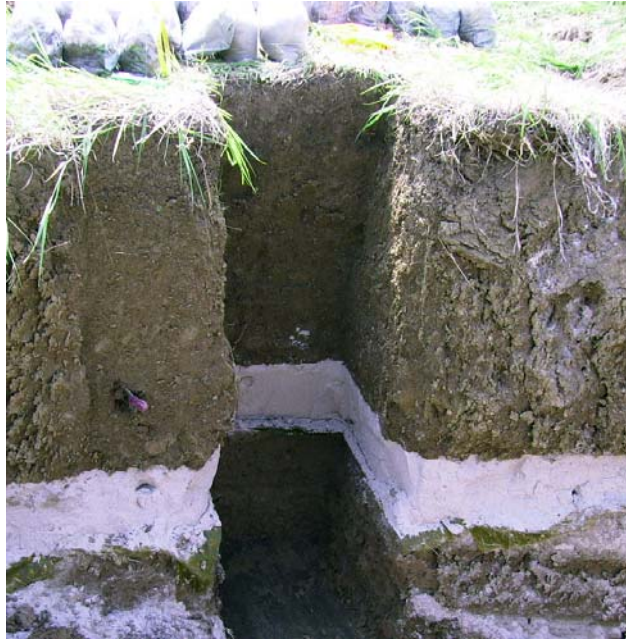
Fig. 6. Near white uniformly graded sand layer used as capillary break in final cover near Omaha, Nebraska (from NUREG CR-7028). Dark layers are fine-textured clay layers used for water storage. Photo after 8 yr of service.
