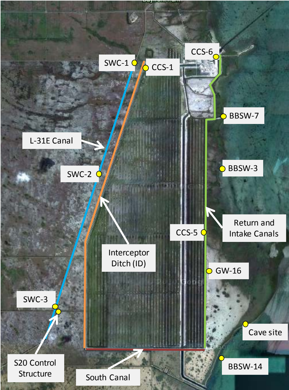
Figure 1: Turkey Point Cooling Canal System showing the main features and monitoring locations mentioned in the text.
