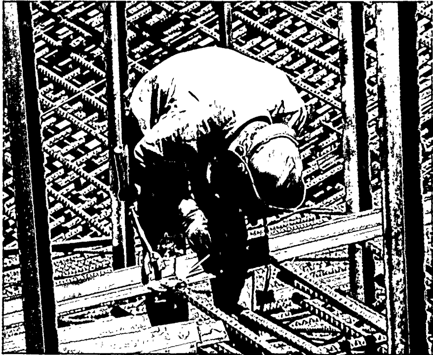
Reinforcing steel was put in place in preparation for a concrete pour at WNP-4.
