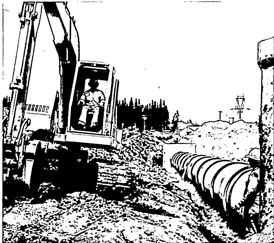
Workmen prepared a drain system to prevent erosion at the WNP-3 and WNP-5 site.
