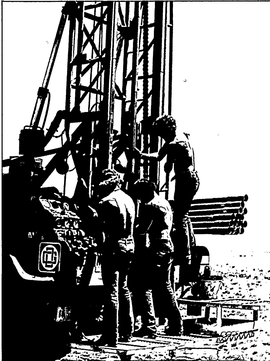
A crew operated a drilling rig in the search for uranium ore in the Red Desert of Wyoming.
