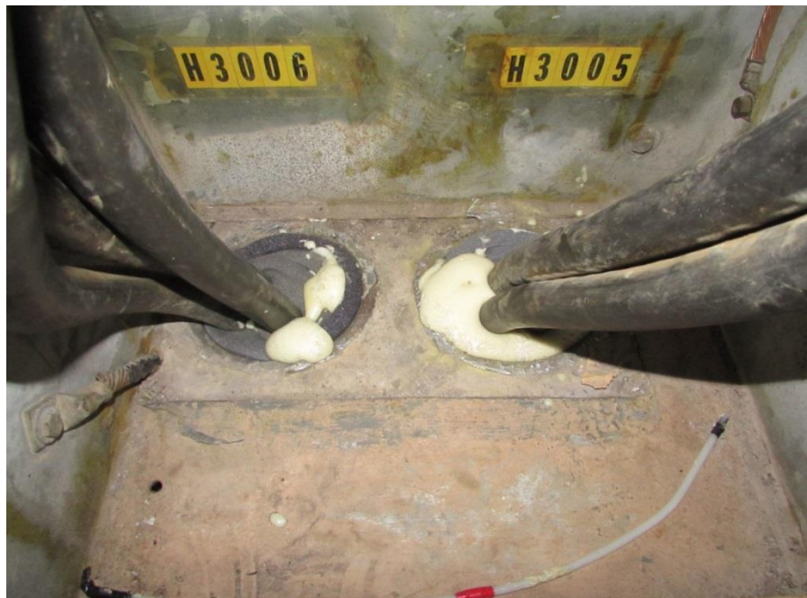
“As-found” (top) and “As-left” (bottom) condition of embedded 6.9kV conduits which penetrate the Turbine and Auxiliary Building at ANO-1. Some of the penetrations are in floors or walls that are flood boundaries.
