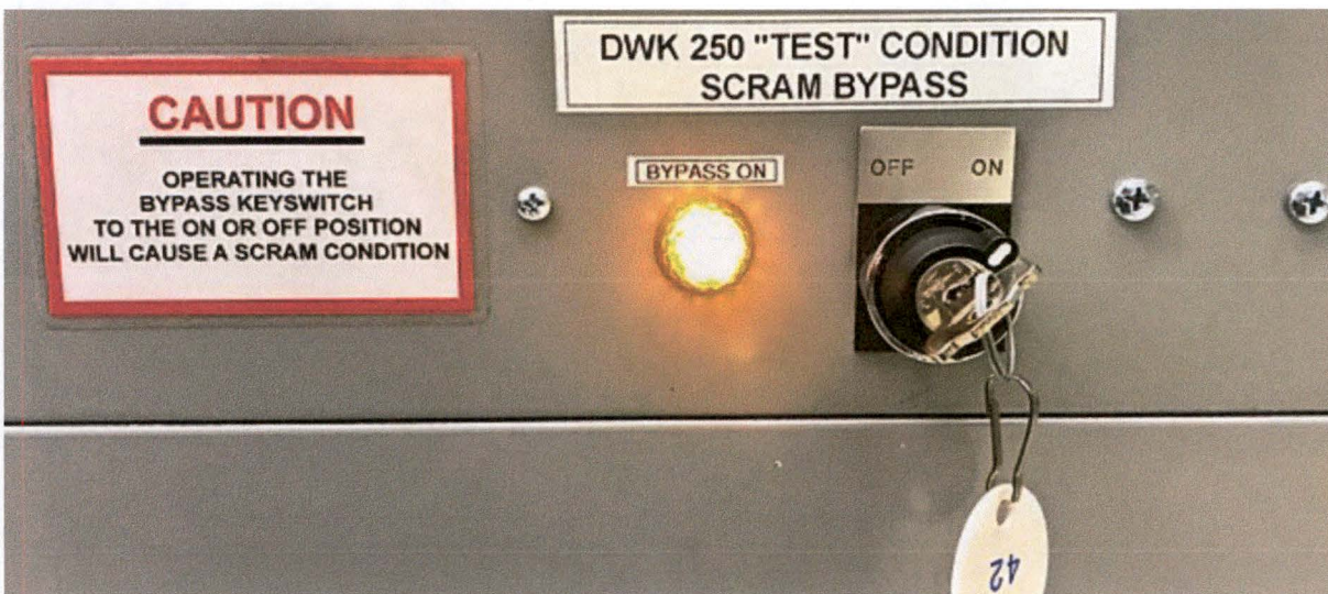
Photo 2 – Front Face of TCB Panel with Caution Posting
