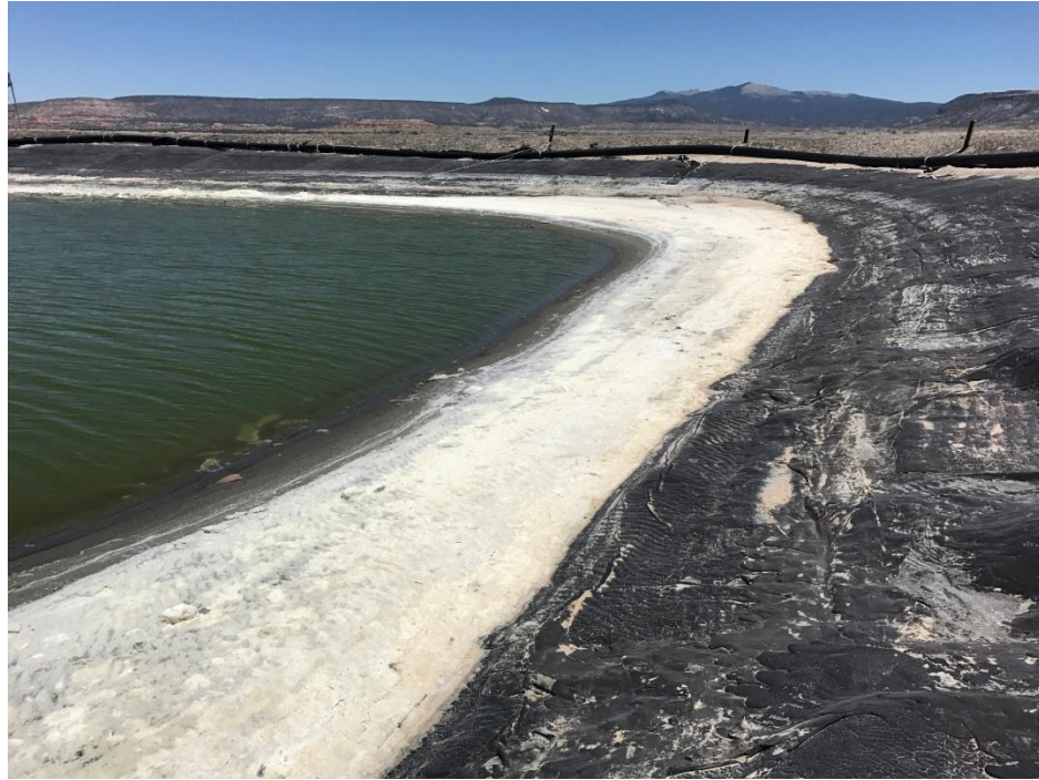
Photo 1 – EP1 liner near the southeast corner. Slumps along right side.
