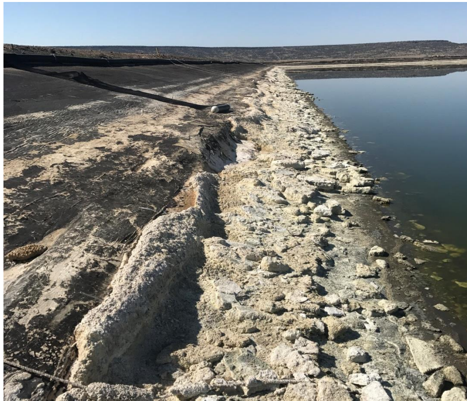
Photo 2 – EP1 east slope. Slumps below normal pool level.
