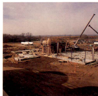
Construction at the Pedricktown site
