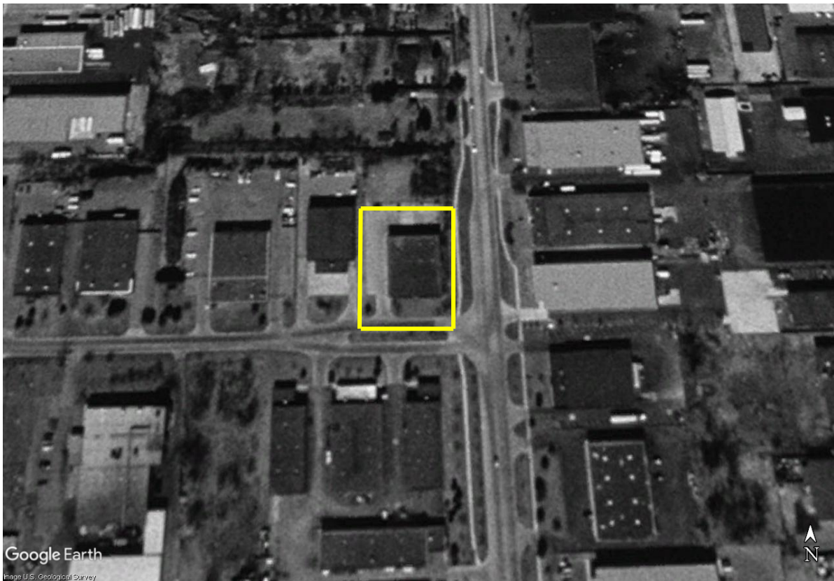
Figure 2. Aerial View of NC Servo Technology (March 1999) (Google Earth Pro 2017)
