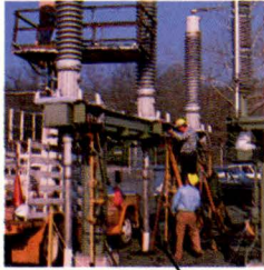
Cable Monitoring System
