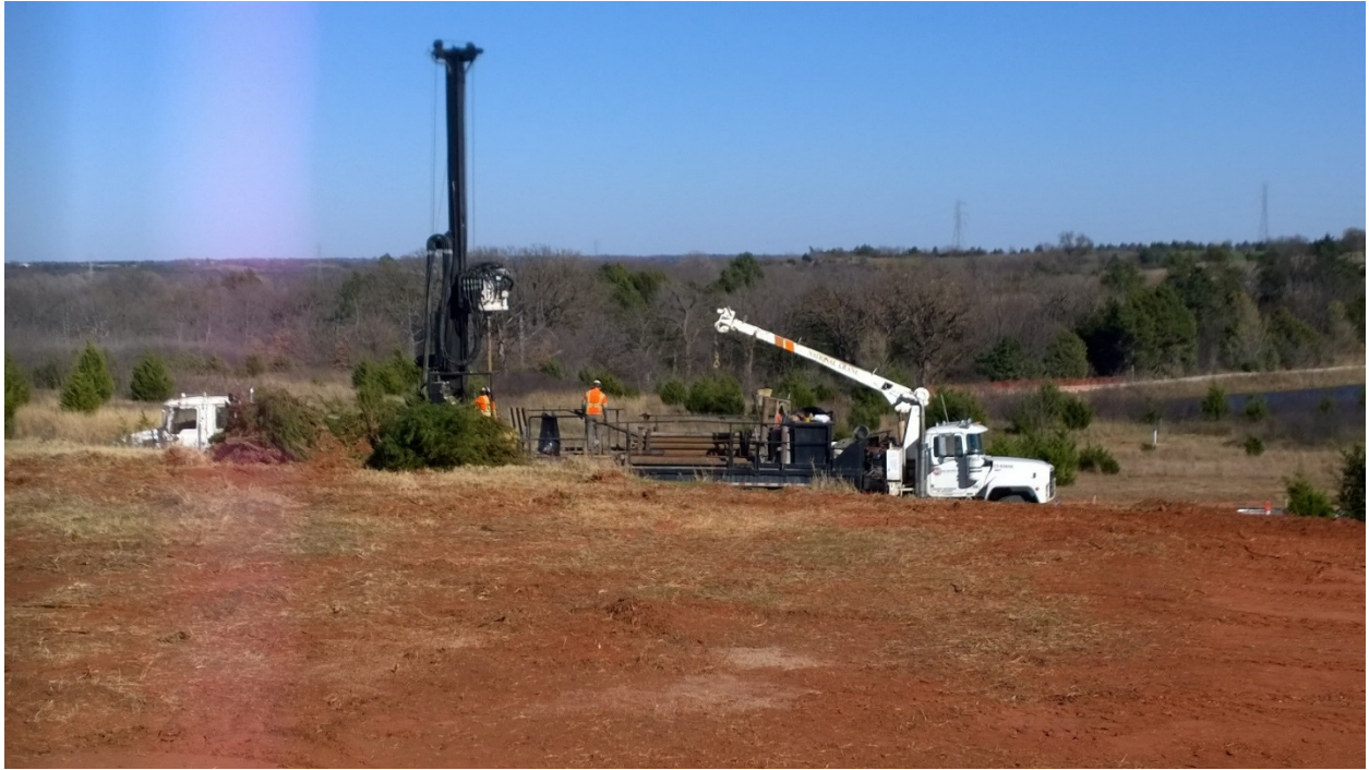
Figure 6: Drilling wells for UP2 area trenches
