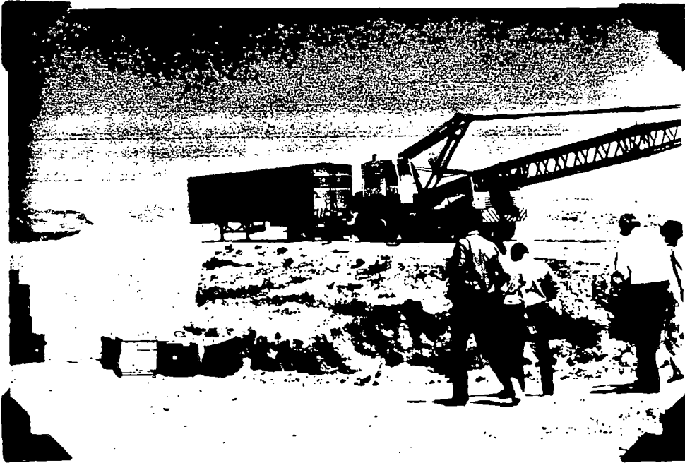
Photograph #5: The relative locations of the Tri-States Trailer and the containers in the trench
