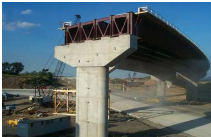
Figure 8. A new overpass under construction in 2001 near State College, Pennsylvania.
