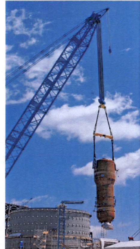
1.4 million-pound steam generator lifted into Unit 3 containment
