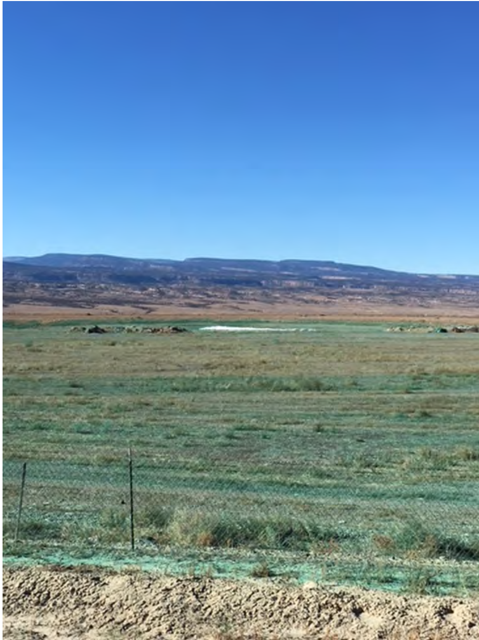
Figure 1: Closed portion of disposal cell with open portion in background
