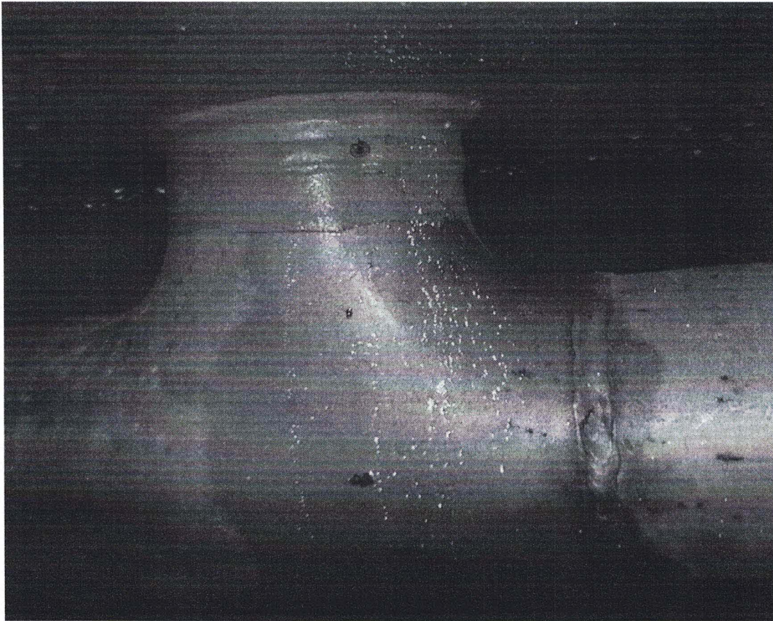
Figure 2 – Pipe Leak at Weld Joint (at top of the tee, in the blue paint)
