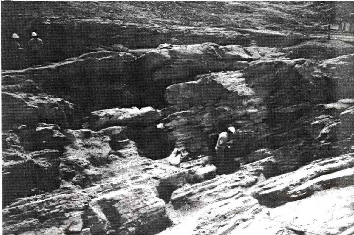
PHOTOGRAPH 26 SOLUTION CAVITIES ALONG BEDDING AND STRIKE-JOINTS ON THE BENCH (EL. 780 FT) ABOVE FACE IV (UPPER), AND KARSTIFIED LIMESTONE IN THE EQUALIZATION BASIN, WITH NUMEROUS CAVITIES
