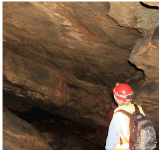
D. Ceiling collapse along bedding plane.
