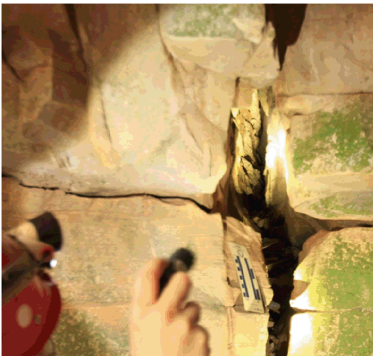
C. Solution enlargement at the intersection of joint and bedding plane
