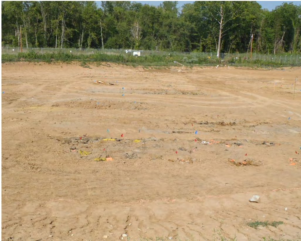
Figure 5 Example of Multiple Burial Pits Visually Identifiable by a Change in Soil Color as Well as by Uncovering Trash and Debris
