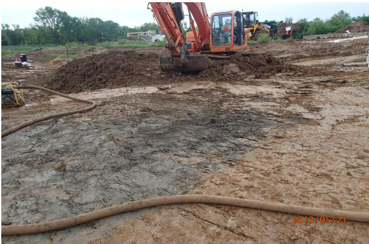
Figure 4 Example of Soil Discoloration where a Burial Pit was Located
