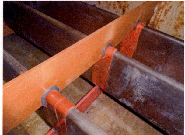
Figure 6: Grommets installed at tape splice location
