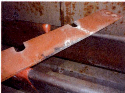
Figure 3: Tracking on bus supports in Non-Critical Switchgear Room
