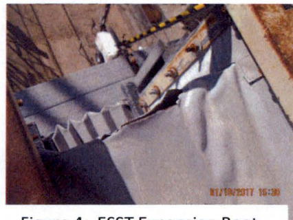
Figure 4: ESST Expansion Boot
