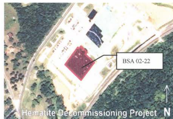
HDP Satellite Site View: See Building 230 in Red Crosshatching
