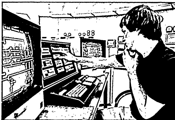
An electronic system of lights and lines on a curved map of the Company's distribution system continuously monitors service and signals when trouble strikes.
