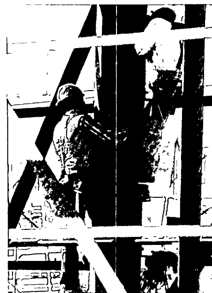
Steelworkers wrestle a girder in place high off the ground as construction continues on San Juan Units 3 and 4.
