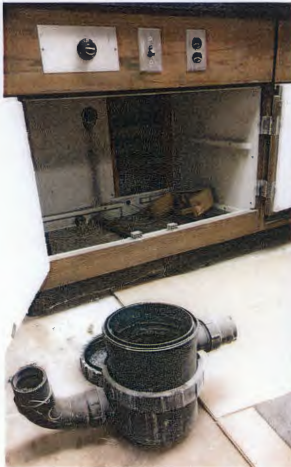
Low-Point for A127 Fume Hood
