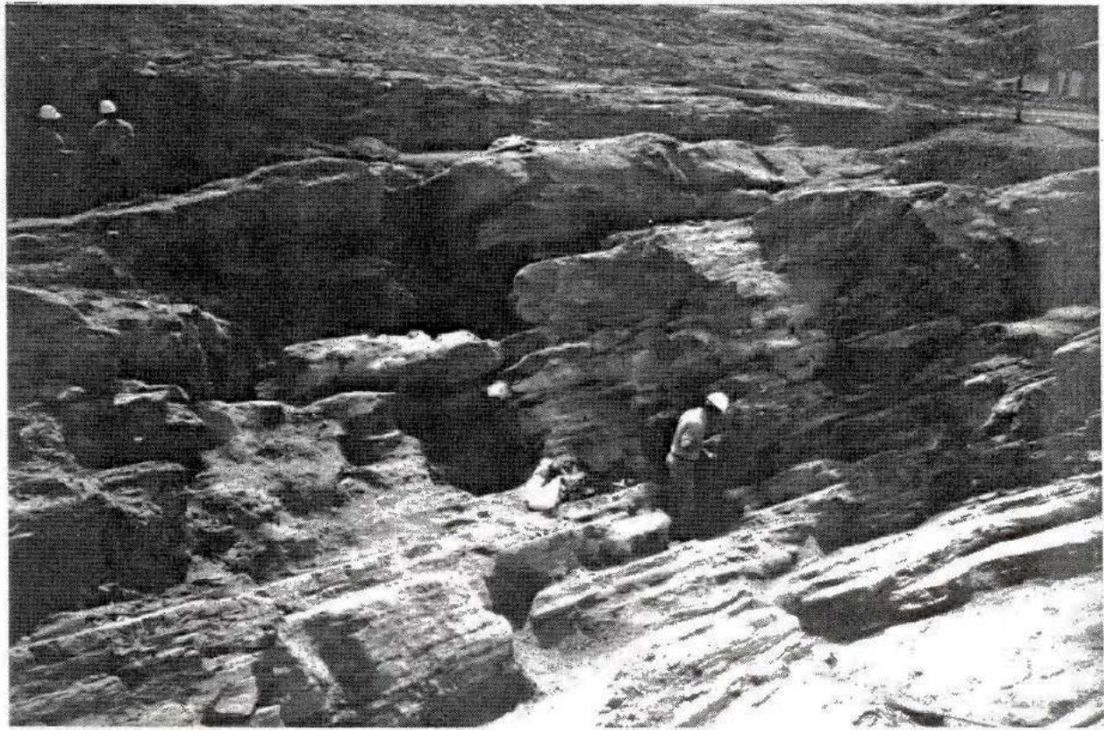
PHOTOGRAPH 26 SOLUTION CAVITIES ALONG BEDDING AND STRIKE-JOINTS ON THE BENCH (EL. 780 FT) ABOVE FACE IV (UPPER), AND KARSTIFIED LIMESTONE IN THE EQUALIZATION BASIN, WITH NUMEROUS CAVITIES
