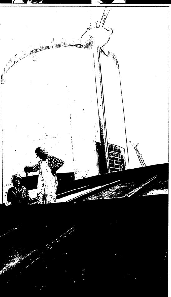
WNP 3 and 5 are duplicate generating plants being built in Grays Harbor County, Washington. The 212-foot-high concrete wall for WNP 3 was placed in a continuous, 21-day pour—a masterpiece of coordination. The work went on around the clock for the full three weeks.
