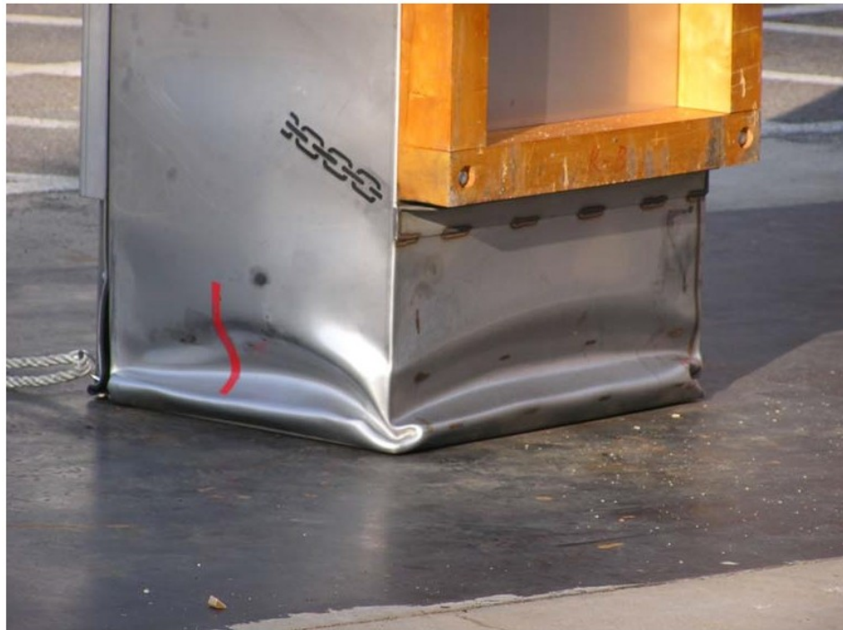
Figure 2-34 Damage from End Impact (Bottom and Side)
