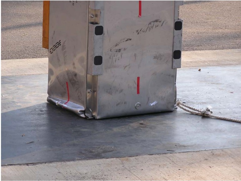
Figure 2-35 End Impact Damage (Top and Side)
