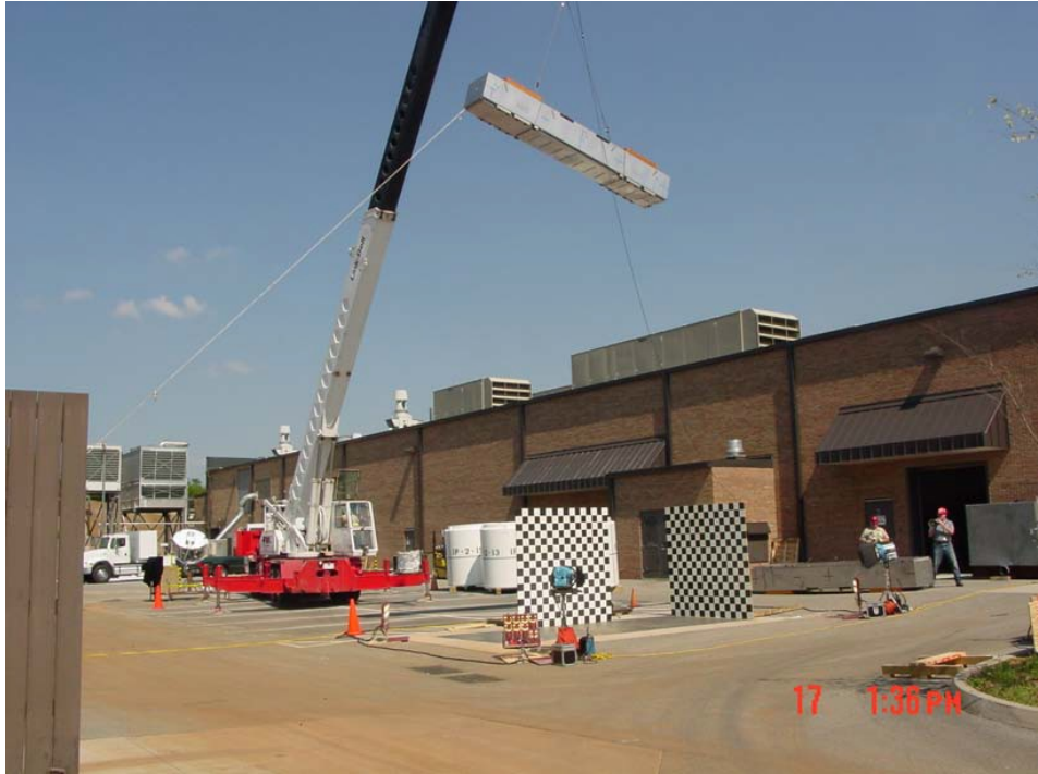
Figure 2-25 CTU 1 Positioned for 15° 9-m (30-foot) Slap-down Drop
