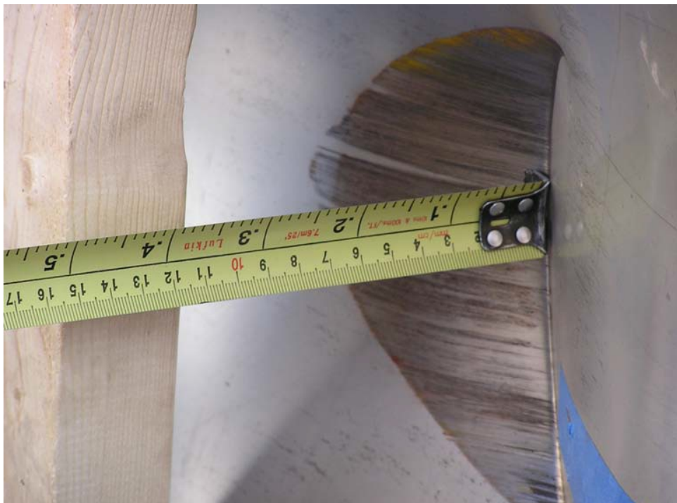
Figure 2-32 Close Up of Puncture Damage
