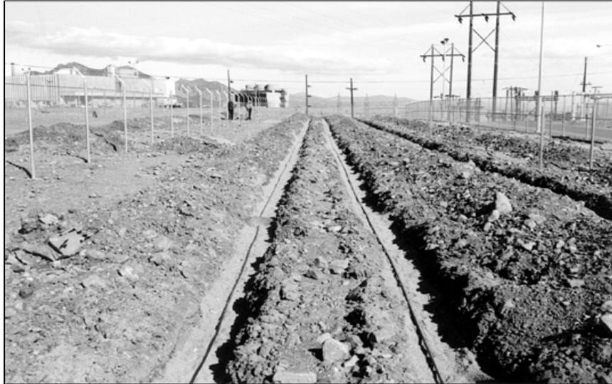
**Figure 20 A typical ported coaxial cable system installation**
