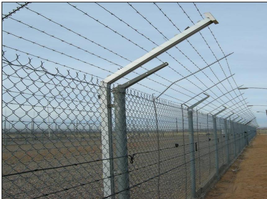
**Figure 27 A taut wire sensor system installed on an existing fence**
