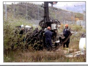
Figure 3-5 Advancement of Core Barrel
