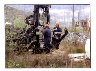
Figure 3-4 Attachment of Core Barrel to Drill Head
