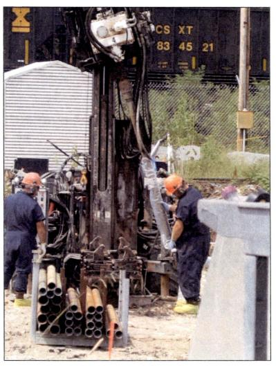
Figure 3-6 Extracting Soil Core from Core Barrel
