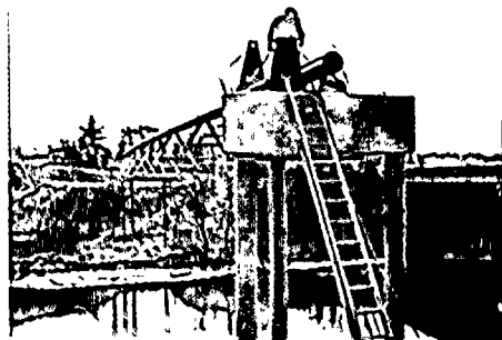
RG&E engineers designed an uncommon type of gas pipeline support in this bridge that crosses the Barge Canal. The support cables are underneath the pipe instead of above.
