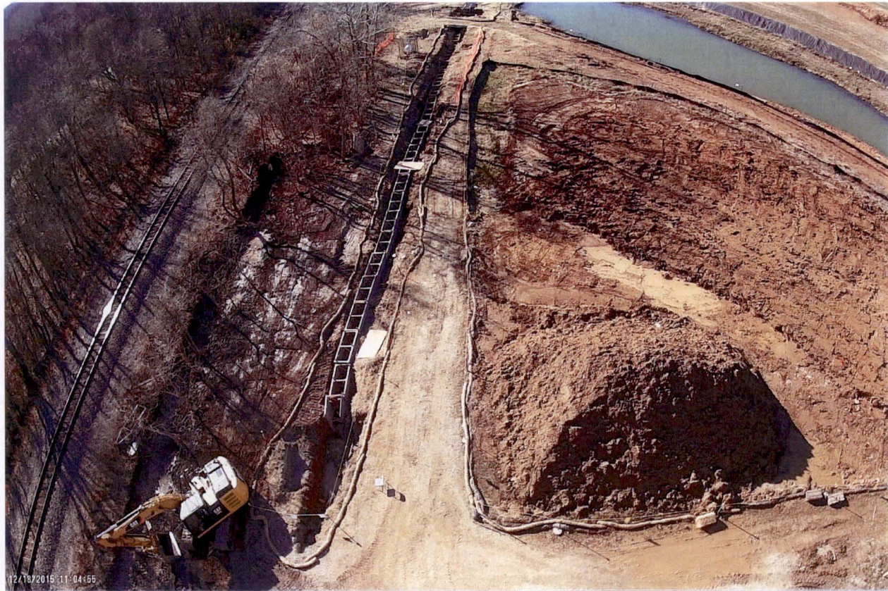
Figure 3-1 SWTP Trench with Trench Boxes Installed
