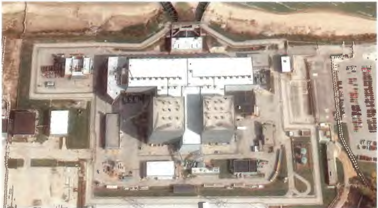
Figure 3.2-2. Point Beach Imagery (Source: Google Earth, 2015)
