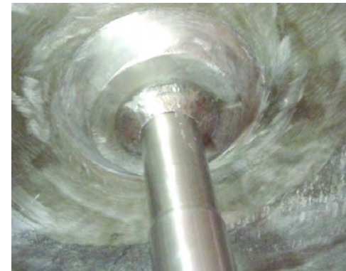
Half-nozzle repairs
