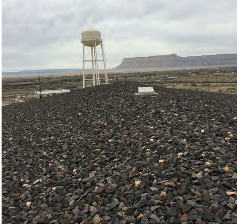
Figure 3: Green River disposal site top of cell with site marker
