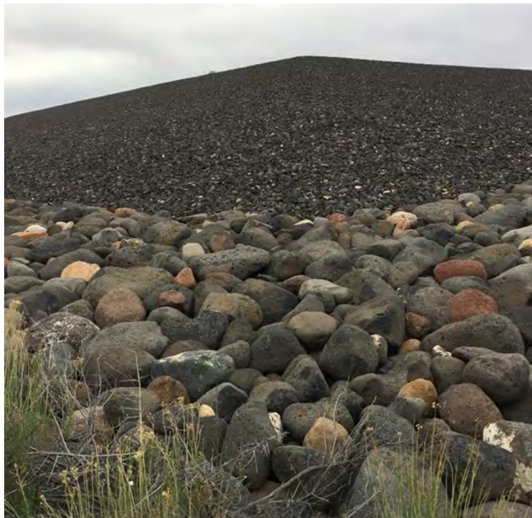
Figure 2: Green River disposal site side slope with rip-rap
