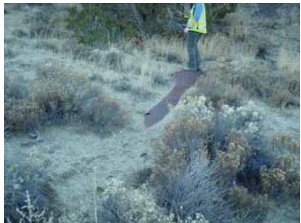
3 ft Metal Culvert (35 ft exposed) Reference Point 32 (11/11/13)
