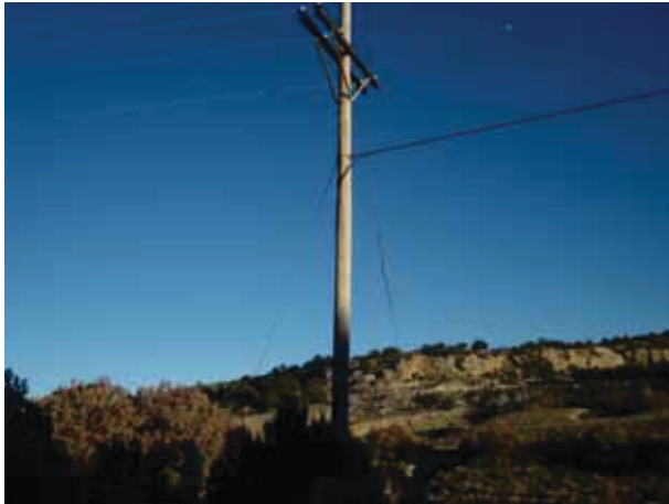
Power Pole Reference Point 24 (11/11/13)
