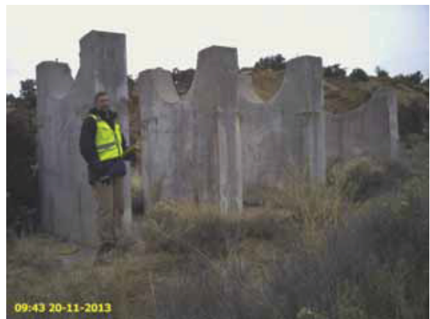
Vent Casing Supports (30ft x 15 ft x 10 ft, pad is 30 ft) Reference Point 73 (11/20/13)
