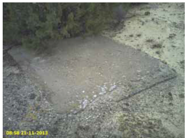
Concrete Pad (3 ft x 5 ft) Reference Point 138 (11/21/13)
