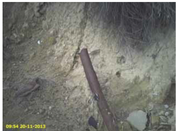
2-inch Diameter Metal Pipes (1 ft and 1.5 ft exposed) Reference Point 79 (11/20/13)
