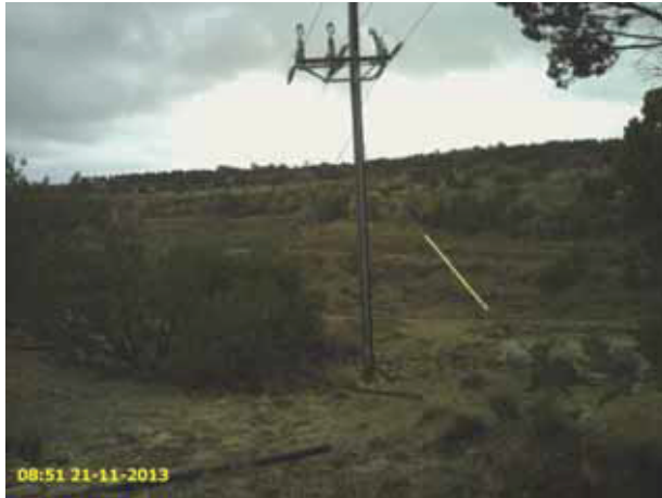
Power Pole Reference Point 132B (11/21/13)
