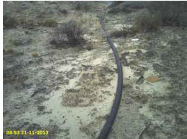
2-inch Poly Pipe (~30 ft exposed) Reference Point 134 (11/21/13)
