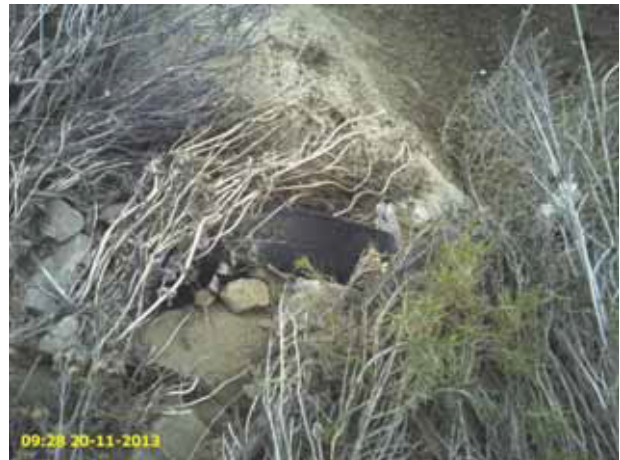
Plastic Pipe (1-ft exposed) Reference Point 65 (11/20/13)
