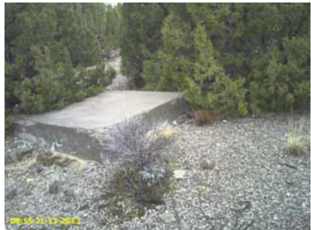
Concrete Pad (3 ft x 5 ft) Reference Point 136 (11/21/13)
