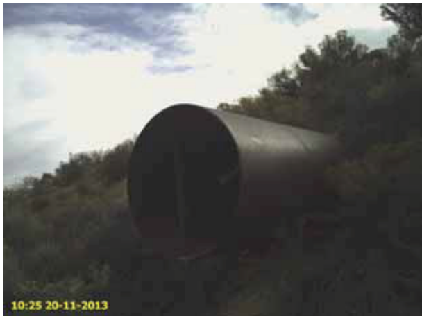
4-ft Metal Culvert Reference Point 100 (11/20/13)
