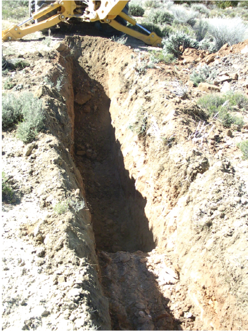
Plate 12: Vent Holes 3 and 8
