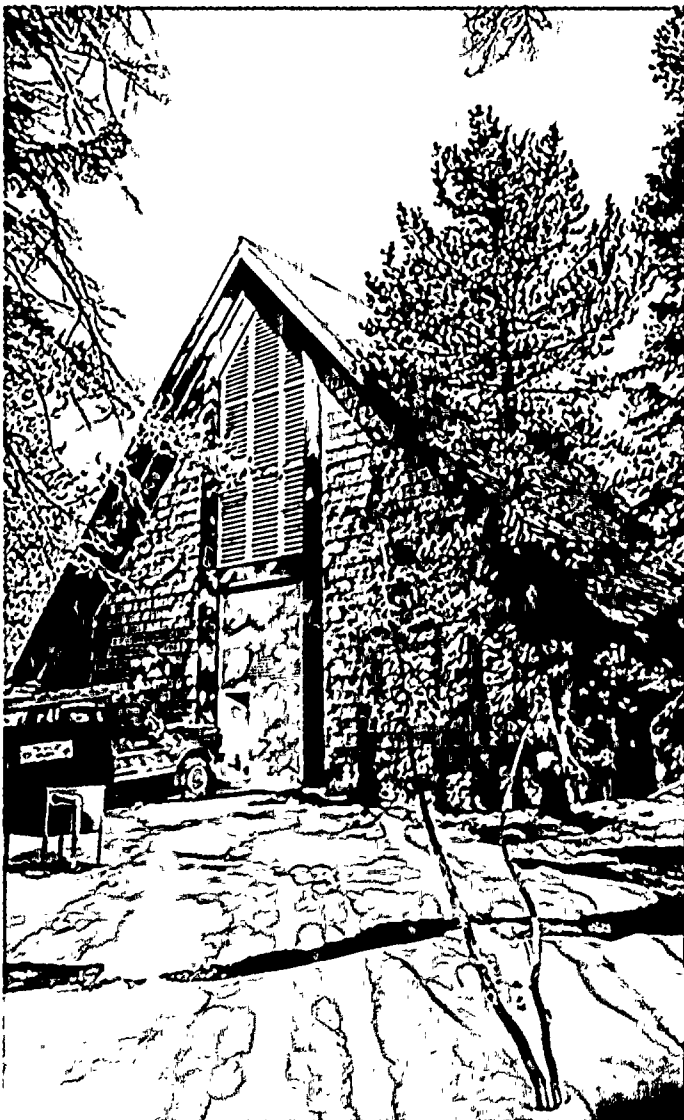
From the highway, this PG&E substation looks like a ski chalet. It serves a big, new, all-year recreational area in the Sierra.
