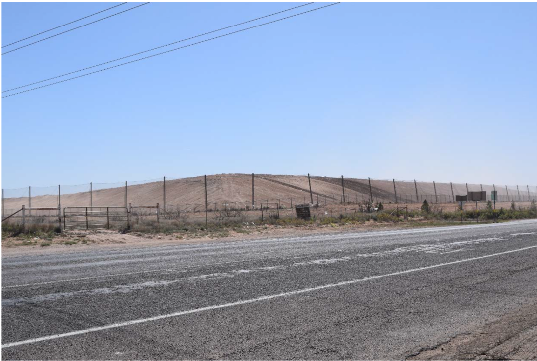
Photo 5b, facing southwest from WCS entrance – foreground range (existing Lea County, New Mexico, landfill).
