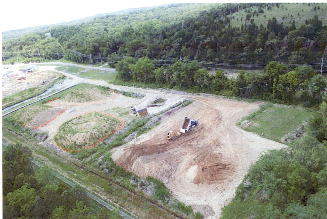
Figure 3-1 Reuse Soil Stockpile Operations – 07/2013
