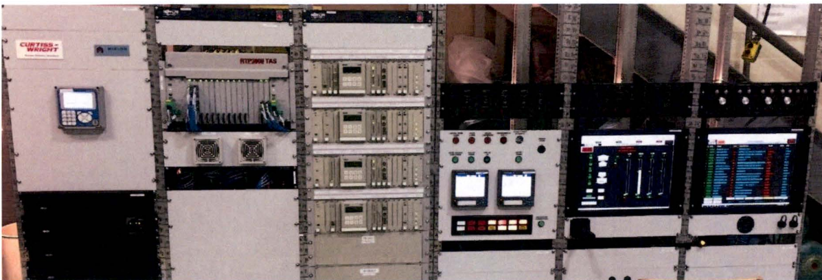
Figure 7-4: Site Acceptance Testing Staging of Reactor Control Console and Display Instruments
