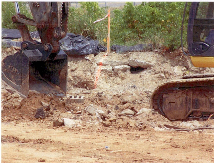
Figure 2-8 Examples of Debris that was Exhumed During Remediation Excavation of the Burial Pit Area
