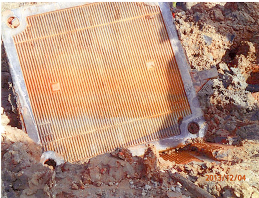
Figures 2-6 Examples of Radium Contaminated Filter Plates Being Unearthed While Excavating in the Burial Pit Area
