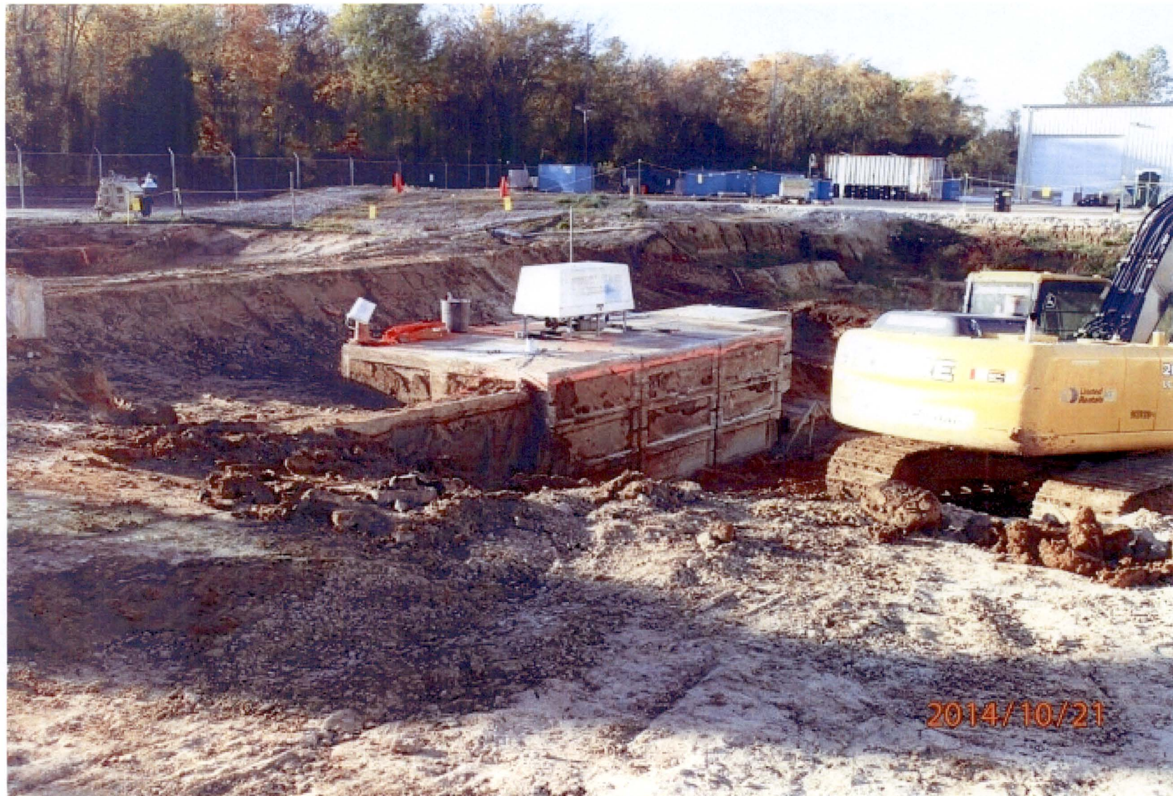
Figure 2-58 Sanitary Wastewater Tanks (Looking SW)
