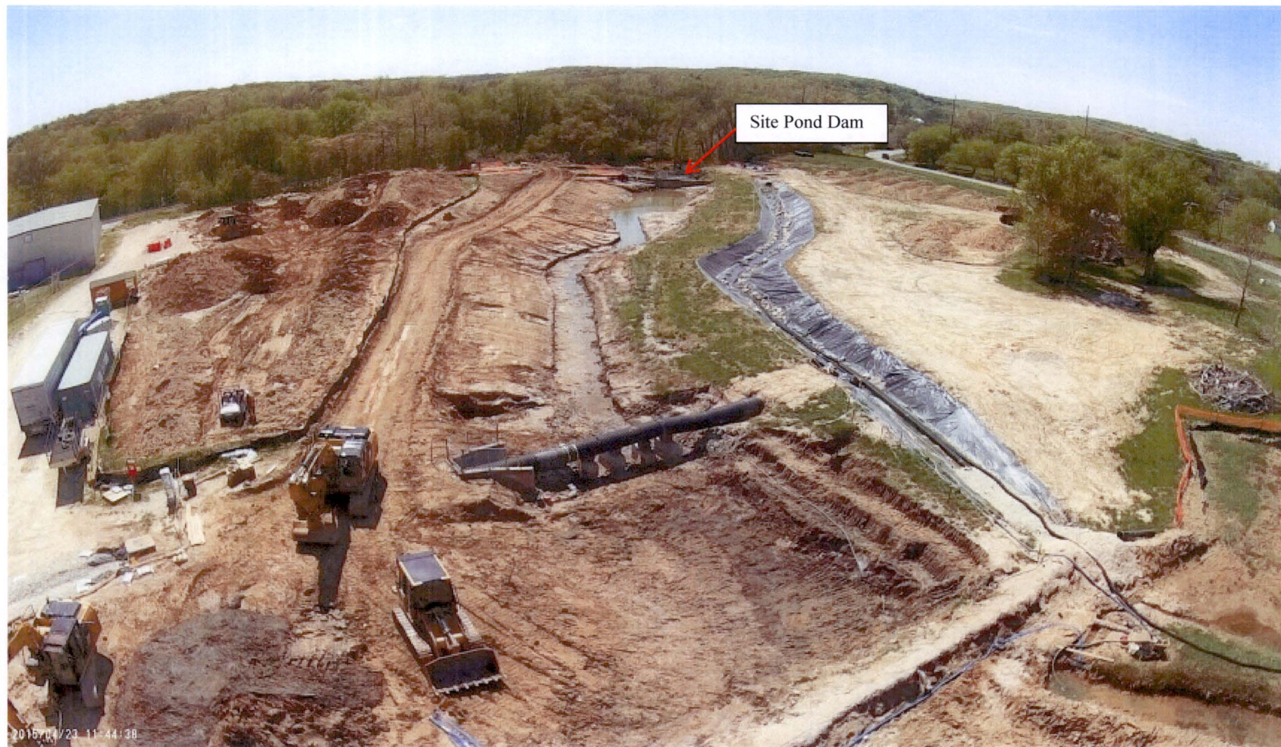
Figure 2-62 Site Pond Excavation and Remediation Nearing Completion (Looking S)
