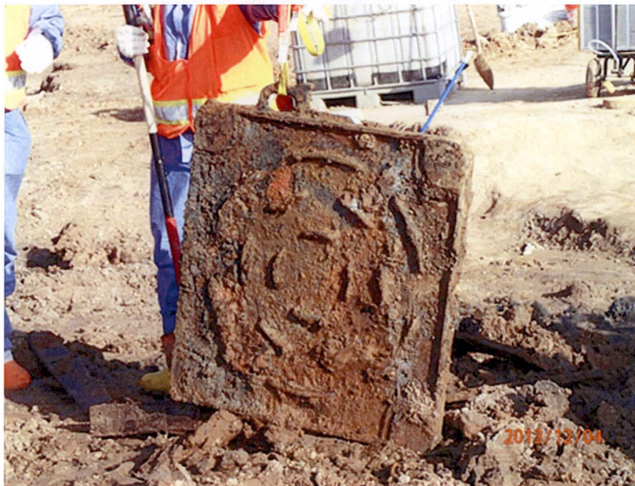
Figure 2-5 Examples of Radium Contaminated Filter Plates Being Unearthed While Excavating in the Burial Pit Area
