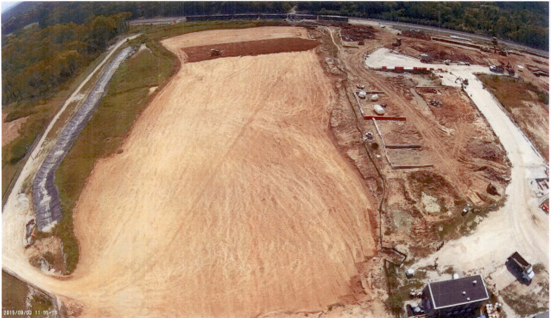
Figure 2-17 Burial Pit Area September 2015 (Looking SE) Backfill Operations in the Burial Pit Area
