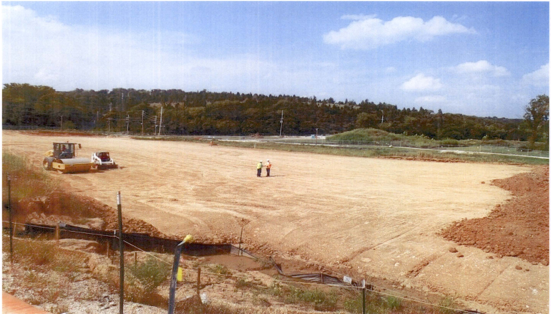
Figure 2-18 Burial Pit Area September 2015 (Looking South) NRC Region III Inspector Inspecting the Backfill of the Burial Pit Area
