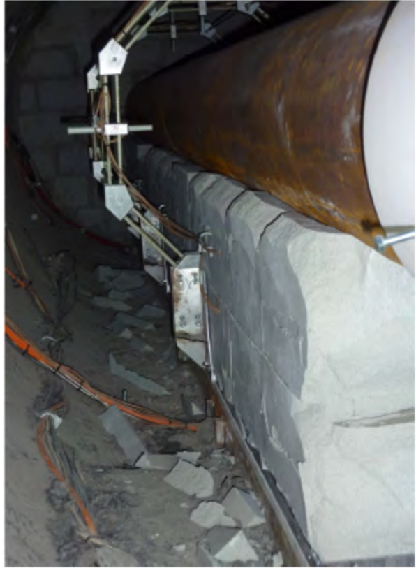
Figure 2-5. Damage to Some of the Bentonite Blocks During the Initial Stages of Construction of the Nagra Section (Teodori and Gaus, 2011)
